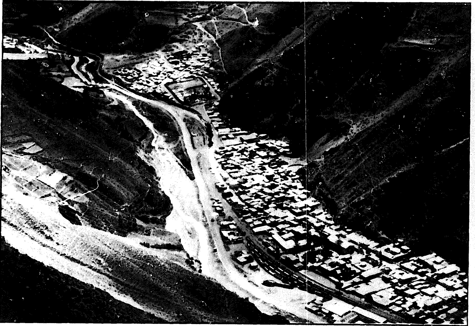
Aerial view of Matucana, Rimac Valley, showing the vulnerable location of the main road, railway and buildings in the floodplain. Erosion is clearly visible on the steep sides of the surrounding mountains, particularly where vegetation cover is denuded.
