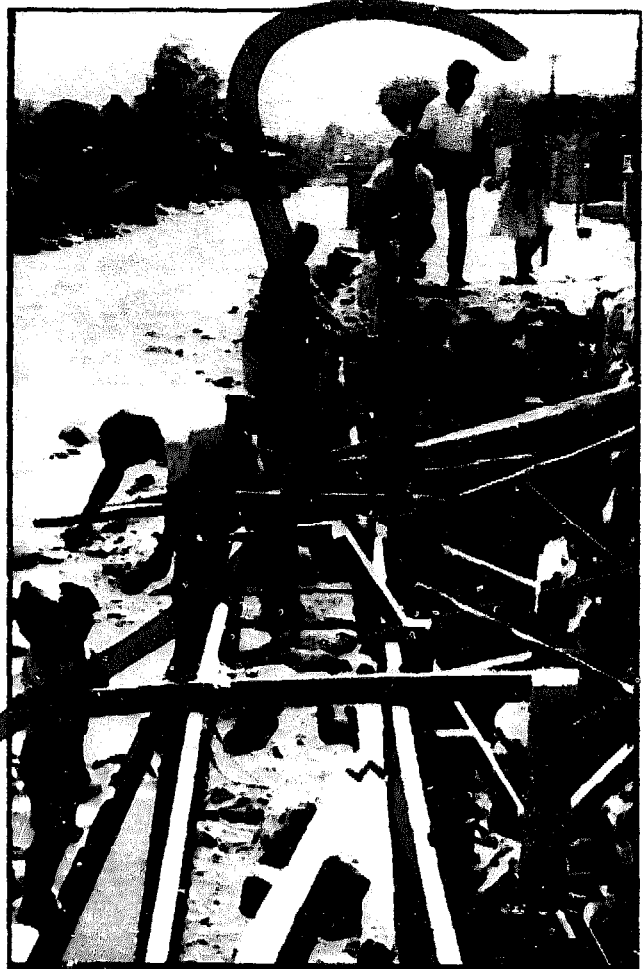
Building river defence walls, Chosica, Rimac Valley. Front cover: Traditional methods and local materials for river defences, Rimac Valley. Photographs Andrew Maskrey/Juvenal Medina/PREDES
