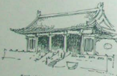
West of the larger buildings in the former Imperial Palace, Beijing, have the roof structure in part supported by huge wooden columns covered with plaster.
