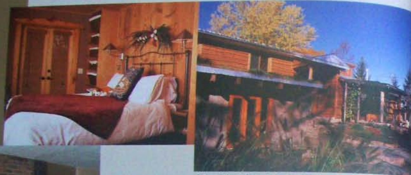
The French doors admit sunlight, while the concrete walls and earth berm block highway noise.
