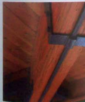
Engineered wood, such as this laminated beam, not only makes efficient use of forest resources but is strong and beautiful as well.
