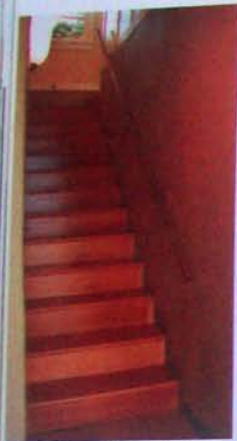
The risers of these Douglas fir stairs were once the treads of the previous (steep) staircase.
