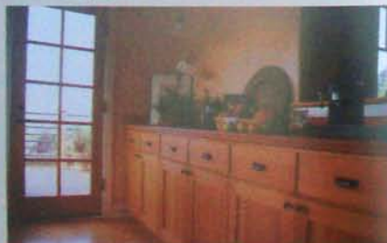
Salvaged Douglas Fir was re-milled to build the doors and drawer fronts of these wheat strawboard cabinets.
