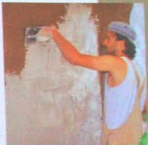
Accomplished earth plasterer Axel Linde led the wall-finishing crew.
