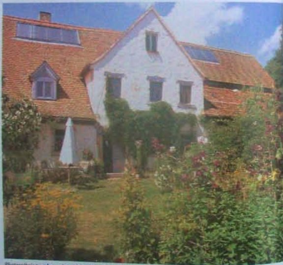
Photovoltaic panels can be integrated into the roof of even historic buildings.
