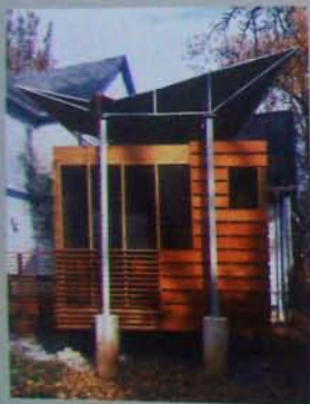
Pier footings minimize damage to the roots of the old nearby tree, and the butterfly roof allows rainwater collection for garden watering.
