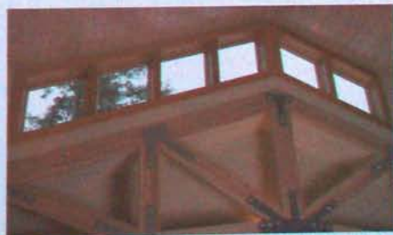
Adding a light monitor with clerestory windows brings reflected light deep into the living space without the liabilities of a skylight.
