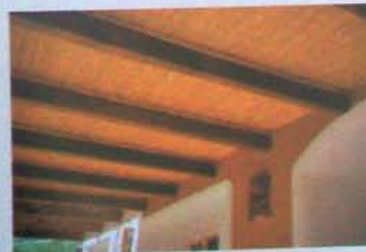
The porch ceilings are of reed fencing, hiding the metal roof and blending well with the other warm, natural materials.
