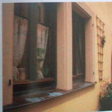
A copper windowsill directs water away from the wall below, protecting it from moisture damage.
