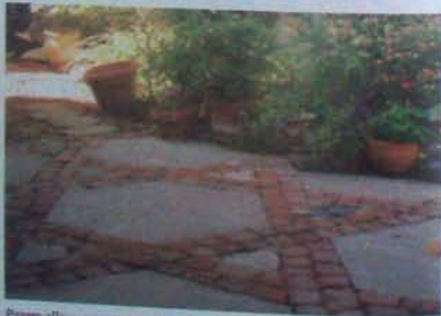
Pavers allow water to percolate into the soil and refresh the aquifer.
