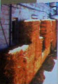
Flashing the house with straw bales.
