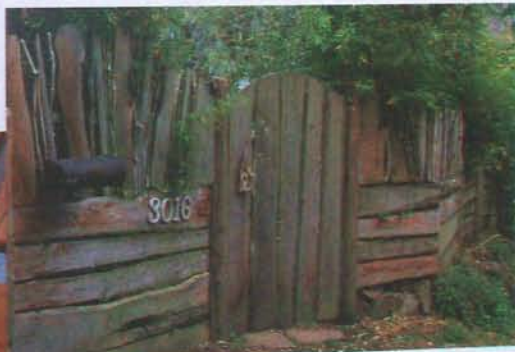
Odd pieces of wood, reclaimed from a lumber mill, were used to build this fanciful fence and entry gate.
