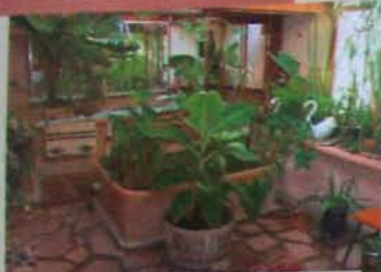
This addition houses a new constructed wetland that processes and cleanses the home's greywater.
