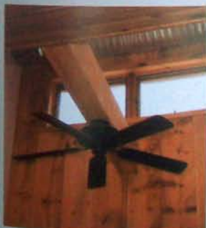
In hot weather, a ceiling fan helps pull warm air up and out through the cupola.
