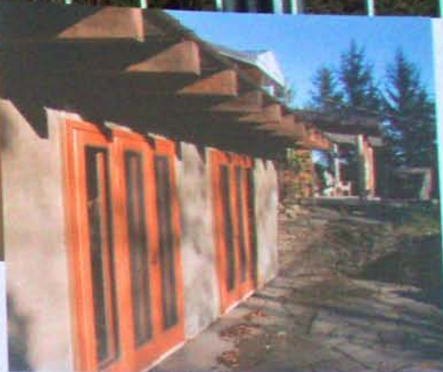
This bedroom addition was designed to increase passive-solar heating for the whole house.
