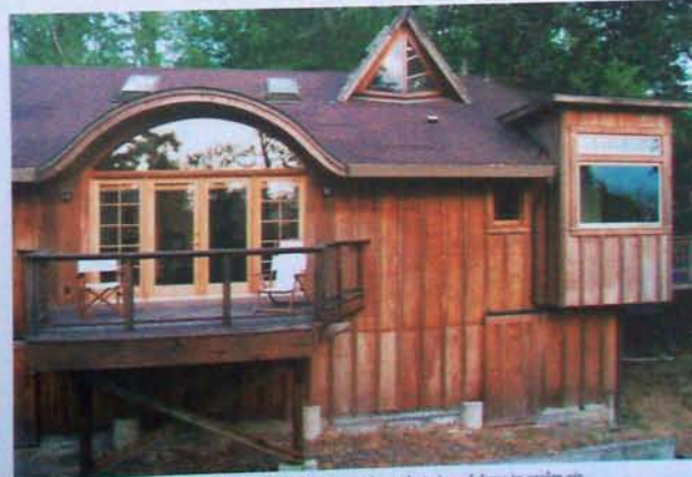
A combination of high and low windows makes it easy to exhaust hot air and draw in cooler air.
