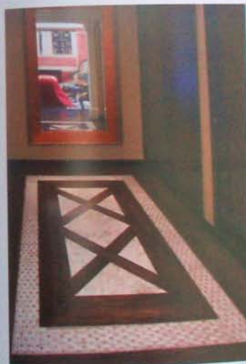
Bringing life in the floor of a short hallway, this classic design is rendered in bamboo flooring and reclaimed marble.
