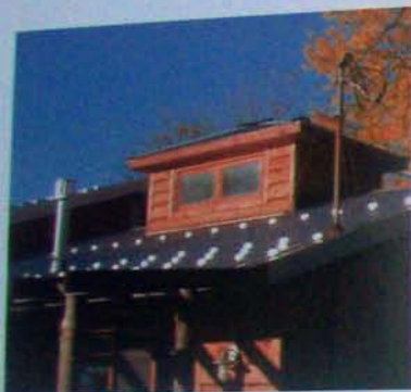
This cabin takes advantage of the chimney effect, naturally ventilating the living space below.
