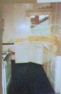
The old basement had stairs, but was too small. Upper cabinets blocked the view of the Goodrich Lake Bridge.
