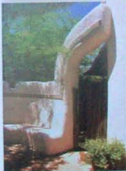
Benches built into the straw bale garden walls provide a peaceful spot to sit and enjoy the surroundings.
