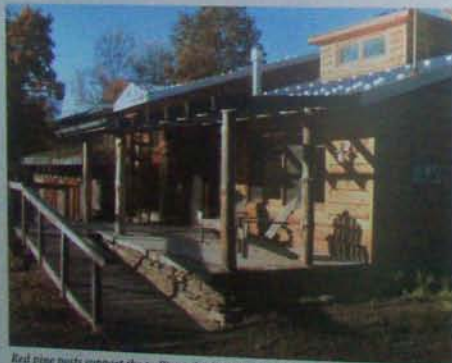
Red pine posts support the trellis at the front of the converted-garage apartment.
