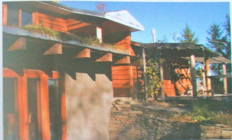
In the summer when the sun is high in the sky, overhangs may keep sunlight from penetrating deeply into a room.
