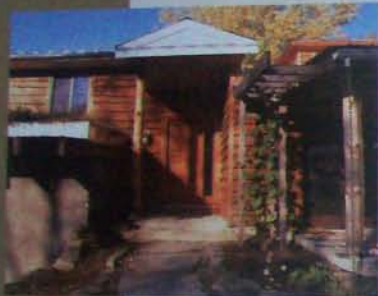
The new entry is much more welcoming; its boldness comes from grain of local red pine, hand-peeled and oiled to carry through the Adirondack look of the siding.
