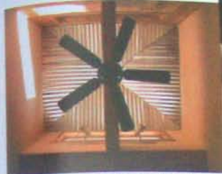
The galvanized corrugated metal ceiling in this cupola reflects light into the apartment below.
