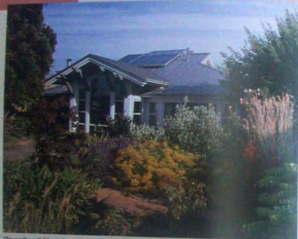
This northern California home integrates photovoltaic panels with a ridge skylight.
