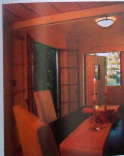
The wide, hinged door that opens the end of this renovated garage was built by carefully deconstructing and rebuilding the previous flip-up garage door.
