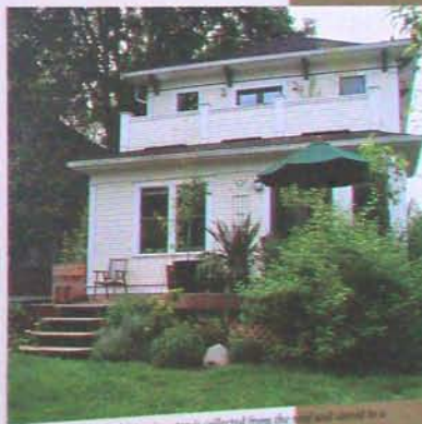
The Northwest's abundant rainwater is collected from the roof and stored in a cistern under the back deck for summer garden watering.
