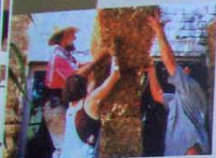
Matts and Judy lift straw bales into place.
