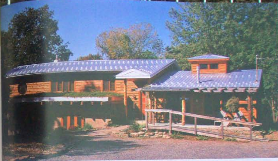
These homeowners reduced their energy costs by overinsulating and employing natural strategies for cooling and lighting.
