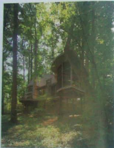
This home was remodelled to bring its owners into greater contact with the natural beauty around them.
