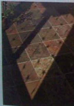
Slate tile on a concrete slab is a good example of thermal mass.
