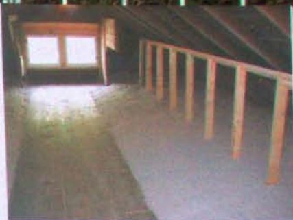
Blown-in attic insulation is fast and cost-effective but doesn't allow the attic to be used as living space.
