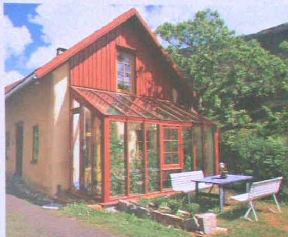
A simple greenhouse addition provides solar heating and a wonderful place for humans and plants to soak up the rays, even on a cold day.
