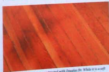
Many subfloors were once constructed with Douglas fir. While it is a soft wood, it ages gracefully and is perfectly serviceable as a finished floor.
