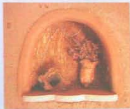
Straw bale walls can easily be curved to create niches.
