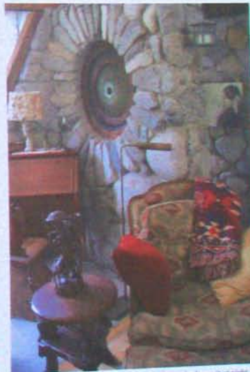
This interior stone wall stores heat during the day and releases it at night when the temperatures drop.
