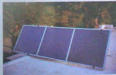
A solar air heater on the roof heats the home in winter.
