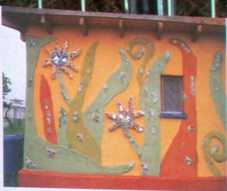
Natural materials, obtained locally, like this brightly colored earth plaster in a bathroom addition in Germany, naturally have low embodied energy.
