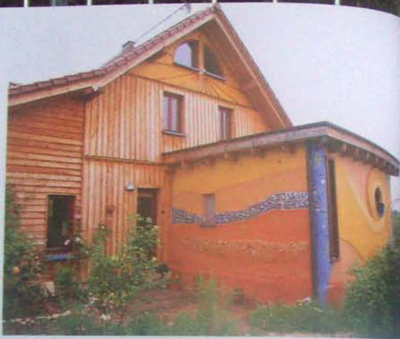
This whimsical earth-plastered addition helps enclose a protected garden.
