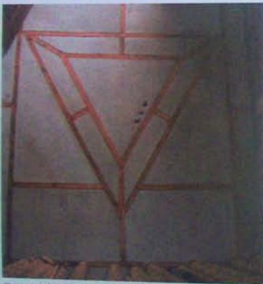
Short recycled studs are used as dividers in this entry floor.
