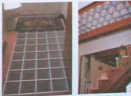
Daylight can be at a premium in townhouses, but the problem is solved here by a translucent panel in the upper bathroom floor, which lets light pass through to the living space below.
