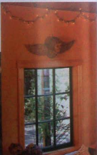
Distributed mass, like this earth-plastered wall, can play an important role in a passive-solar heating strategy.
