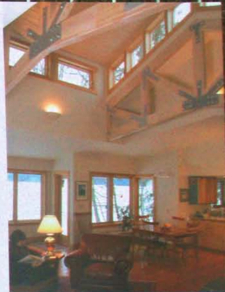
Bringing sunlight into this formerly dark ranch house was a primary goal for this remodeling project.
