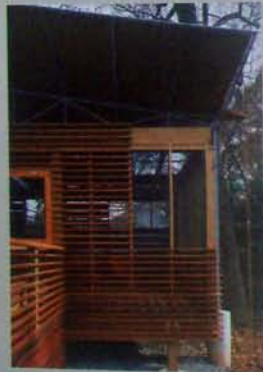
These slats are narrower and the spaces between them wider, allowing more air and light to pass through where privacy isn't needed.
