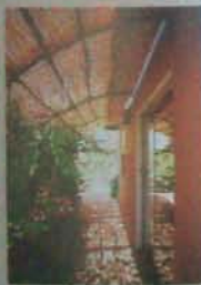
A patio roof made of reed mats can turn the hot western side of a house into a comfortable shade garden.
