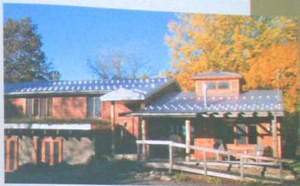
The original garage became a wheelchair-accessible in-law apartment, complete with a trellis front porch and a well-integrated ramp.
