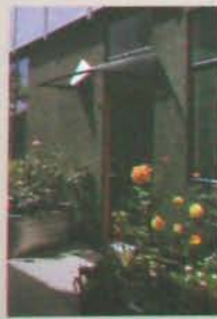
In a whimsical expression of recycling, a used Mazda hatchback window provides an entry roof.
