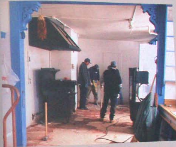
Construction is messy and disruptive, even in the best of circumstances.
