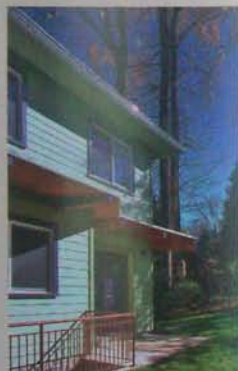
Roof overhangs on the first and second floors provide shade to help keep the addition cool in summer.
