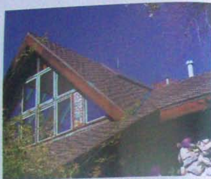
This California home owner added operable windows to draw out hot air in summer.
