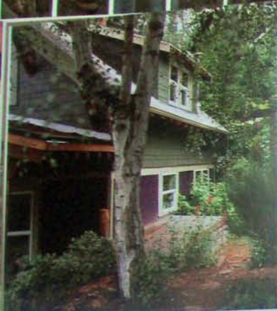
Older wood siding and trim can be rejuvenated with caulk and a colorful paint job, as in this Portland, Oregon, home remodeled by Bloom Design.
