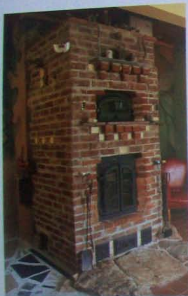
High-mass masonry stoves burn a fast, hot fire to heat the thermal mass, then radiate heat for many hours.
