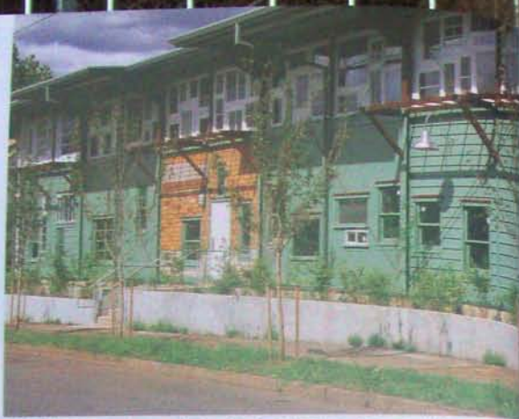
The ReBuilding Center used an array of salvaged windows and siding when they constructed their new building in 2005.
