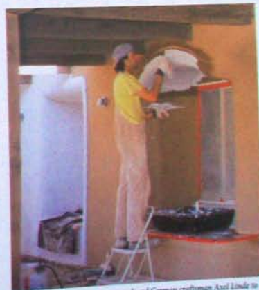
Matt Myrman and Judy Knox employed German craftsman Axel Linde to oversee the earth-and-lime plastering of their house.
