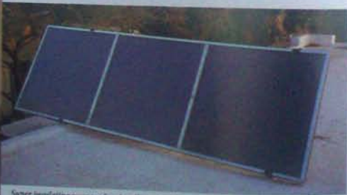
Super-insulating your roof and walls and including a solar hot-air collector may provide all the heating you need.
