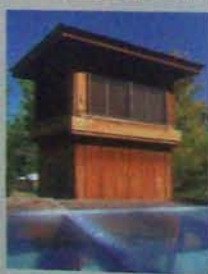
Breezes are cooled by passing through the damp pads of the evaporative cooler at the top of the tower, then drip down into the greenhouse, cooling it by an average of 12 to 15 degrees.
