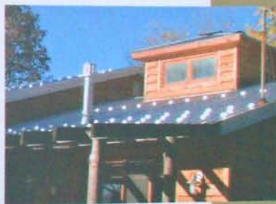
The cupola not only adds visual charm, but also provides natural light and ventilation.
