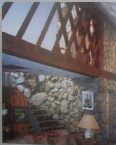
A salvaged bridge truss supports a new second floor, while adding a feeling of visual interest and timeless solidity to this living room.
