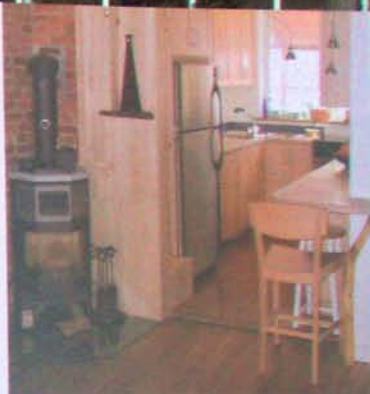
Place your wood stove next to a thermal mass wall. It will store heat and continue to radiate it even after the fire is out.
