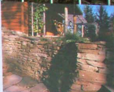
Together with a local mason, Brent and Diana were able to do much of the labor involved in laying their dry-stacked stone walls.
