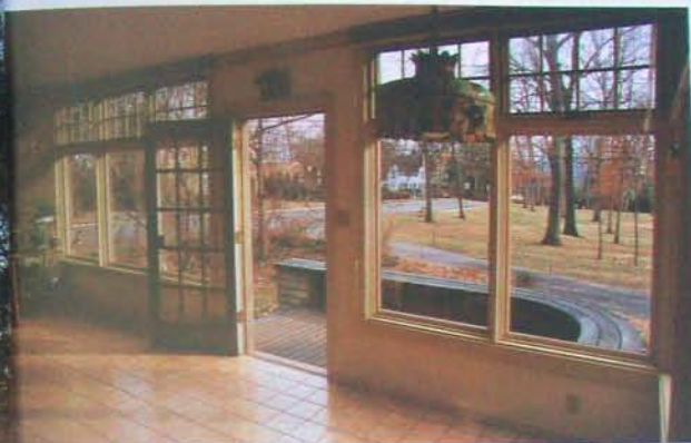
This thermal mass floor soaks up the day's solar warmth and radiates it to the room's occupants as the air cools. Large windows admit plenty of light and connect the room to the outdoors.
