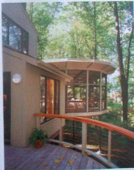
An elevated screened porch on a Virginia house extends the living and dining area into the forest. In this hot, humid climate, shade and breezes are crucial to natural summer comfort.
