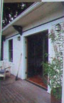
Lots of natural ventilation and shading are all the summer cooling you really need in Portland's mild climate.
