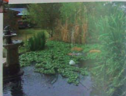
Exiting the interior constructed wetland, the water flows into an exterior rock marsh, where it is further cleaned by cattails, river reed, bulrushes, and other aquatic plants before entering the adjacent evaporative pond.
