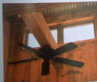
High operable windows meet two goals: natural lighting and stack ventilation (aided by a ceiling fan).
