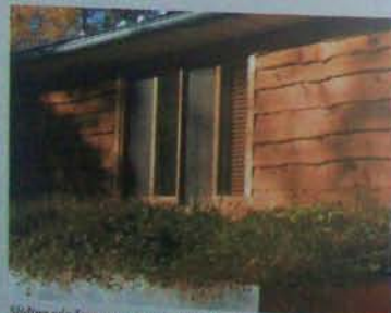
Sliding windows now open to allow the Katzmans to pick herbs and strawberries from the "green roof" of the downstairs addition.
