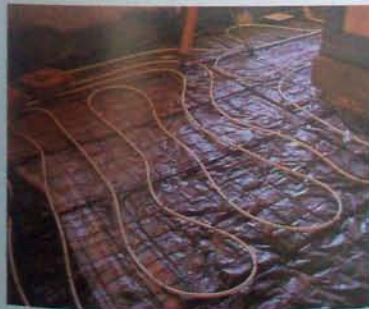
Tubing for hydronic heating systems can be mounted between existing floor joists or laid down before pouring a new concrete slab.
