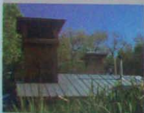
An updraft solar chimney tower is coupled with a slanted evaporative cooling tower to passively cool the greenhouse during the summer.
