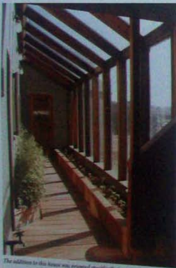
The addition to this house was oriented specifically for passive solar heating.
