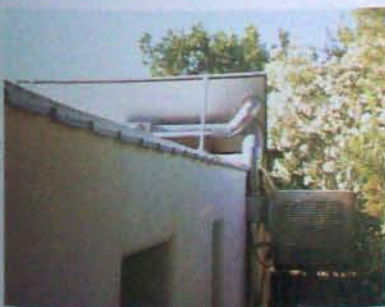
In a climate with hot, dry summers, a swamp cooler (far right) can replace an air conditioner, at a lower operating cost.
