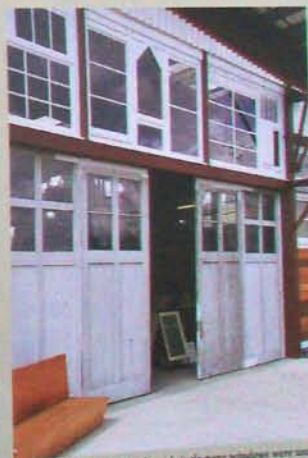
At the ReBuilding Center, salvaged single-pane windows were used to bring daylight into the open-air warehouse.
