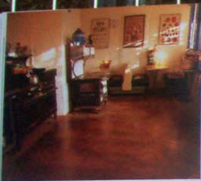
Stained with ferric sulfate, this concrete floor is smooth and durable. The space is heated via hydronic tubing in the floor.
