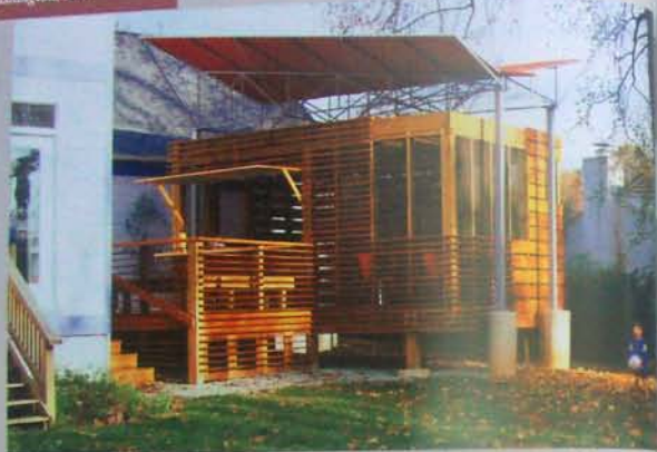
The Rapaports' outdoor room is open to sunshine and breezes, and screened to keep out insects. It stands away from the house so as not to shade the indoor rooms.
