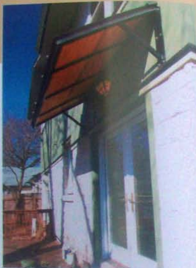
Simply adding an awning over a window or glass door can make all the difference when the summer sun heats down.
