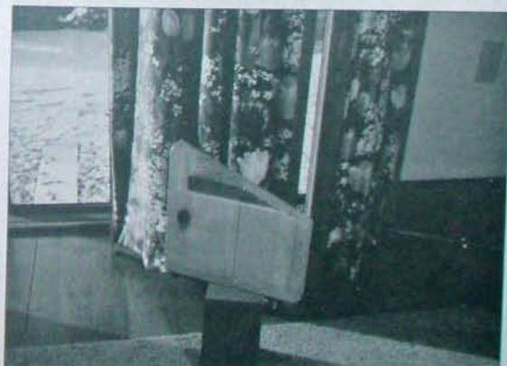
Detail of thermo-shutter showing use of curtains as decorative finish. When in the open position, the folded-back shutters are no more obtrusive than curtains along the sides of a window or glass door. Likewise, when closed, the window will appear to be covered by curtains, yet the insulation value of the layered shutter is far superior to that of curtains alone.
