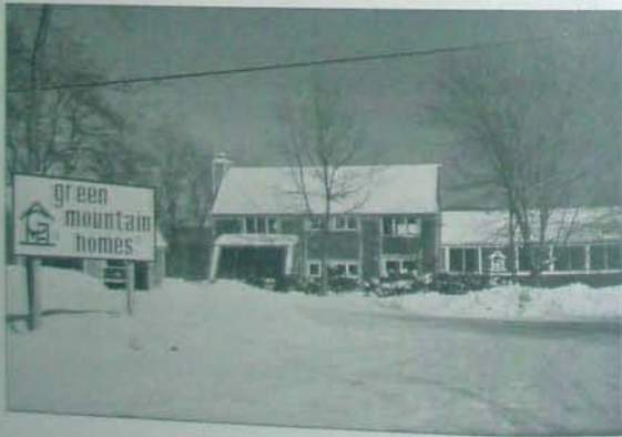
The Green Mountain Homes factory practiced the lessons we preached: the building where our houses were fabricated was itself solar-heated, energy-efficient, and largely lit by daylight.
