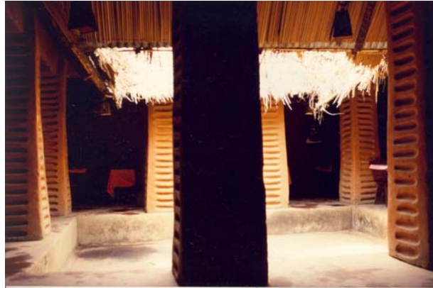
Figure 1 Surface stabilisation of soil with palm oil, Nigeria
