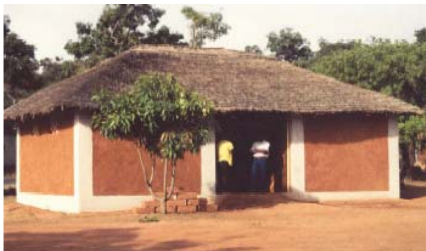
Figure 4: Demonstration house in Jos, Nigeria, built with adobe laid in mud mortar and plastered with mud mortar ©CRATerre/EAG
