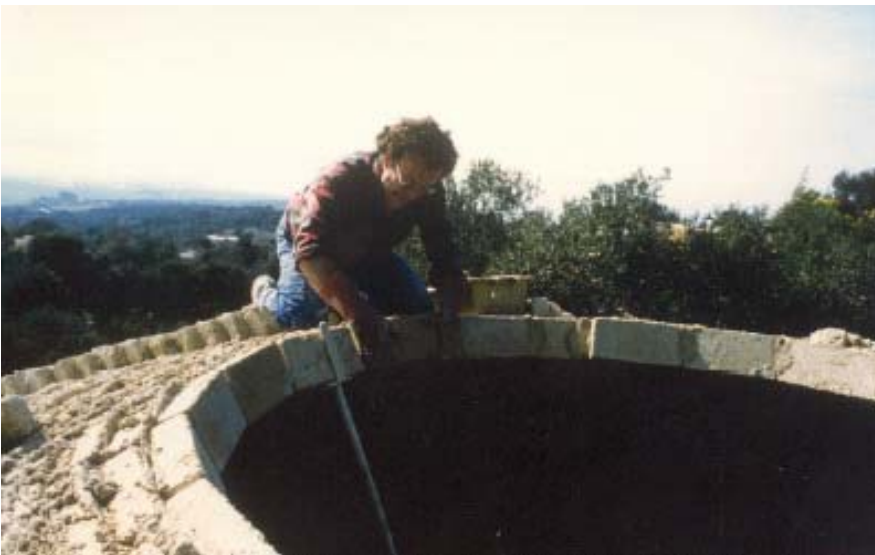
Figure 2: The good cohesion of mud mortar allows construction of vaults and cupolas without shuttering. CRATerra-EAG
