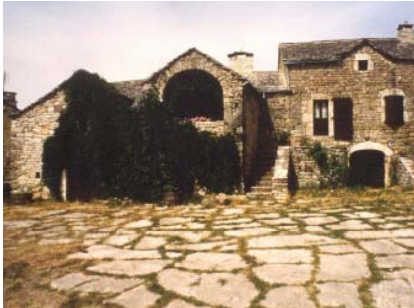
Figure 1: House, Built of stone laid in mud mortar with paving stone yard of stones in mud mortar ©CRATerre/EAG
