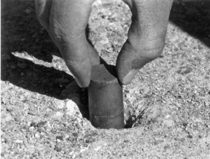
Figure 6. Automatic steering control system uses magnetic markers buried along the center of the lane 1.2 m apart. Photo by Gerald Stone, California PATH.
