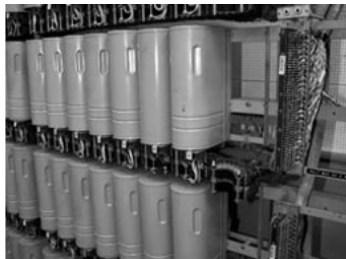
Figure 7. A bank of step-by-step switches used in a telephone central office.
