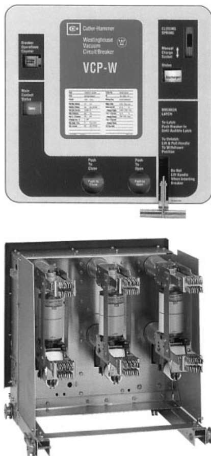
Figure 5. Removable vacuum breaker (2). Reprint-Permission by Cutler-Hammer.
