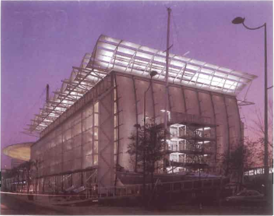
Figure 19 The British Pavilion, Expo '92. © BP Solar. Reprinted with permission.
