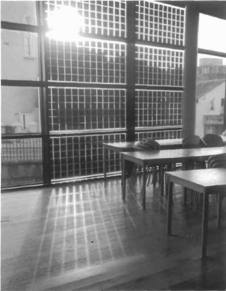
Figure 9 William Jefferson Clinton Peace Centre PV facade, Enniskillen, Northern Ireland, UK.
