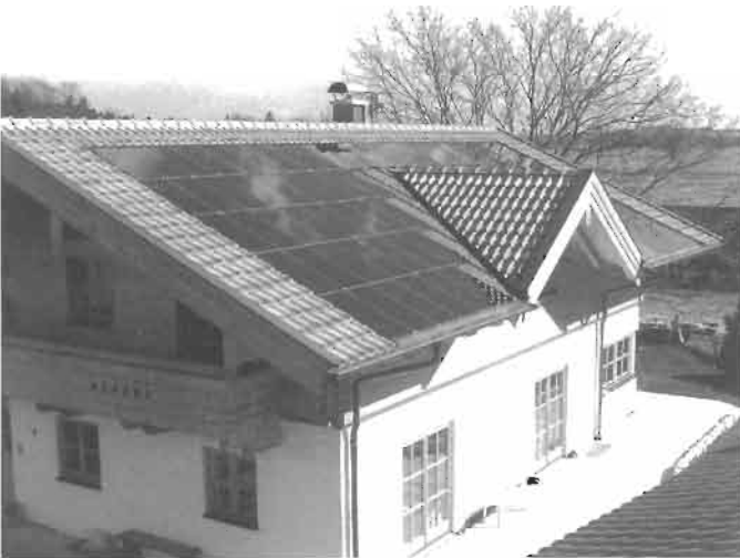
Figure 27 Installation of CdTe modules on a private residence roof.
