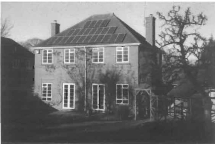
Figure 2 Domestic PV systems for Mr. Treble, Farnborough, UK.
