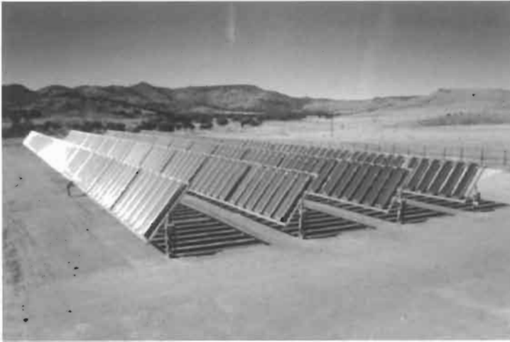
Figure 18 Example of an array field: 100 kW system at CSW Solar Park in Texas made by ENTECH Inc. The plant is composed of four arrays. Each array comprises 72 refractive Concentrator Modules with 220 m 2 total aperture. (Courtesy of Entech Inc.)
