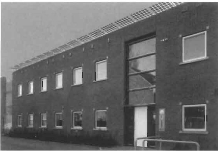
Figure 4 Flat PV roof at Gouda. (© BEAR Architecten. Reprinted with permission).
