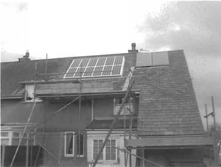
Figure 5 PV retrofits for New Progress Housing, UK.
