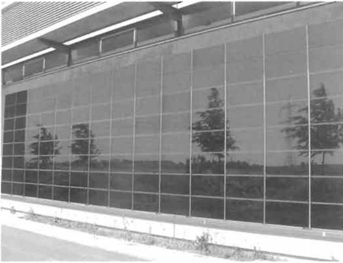
Figure 26 Installation of CdTe modules from ANTEC Solar on the wall of a public administration building.
