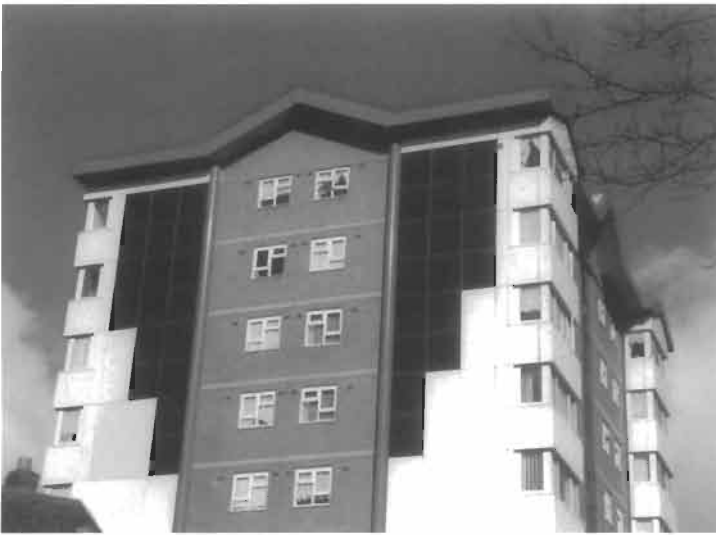
Figure 8 Bowater House PV facade, Birmingham, UK.
