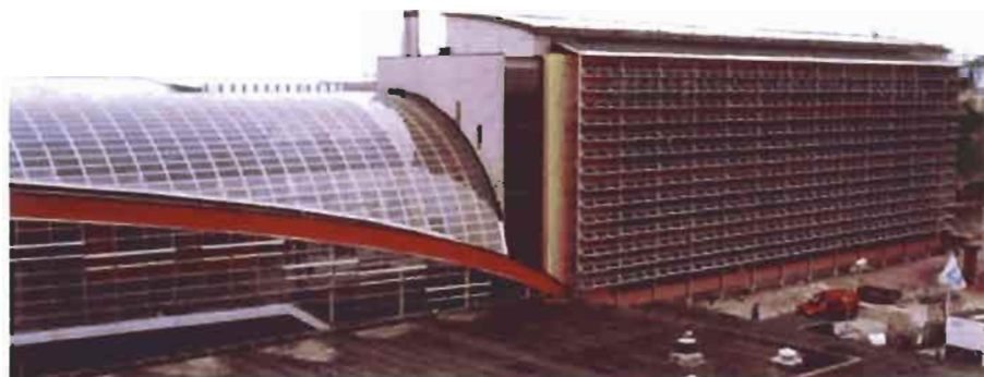
Figure 20 ECN, Buildings 31 and 42. © BEAR Architecten.
