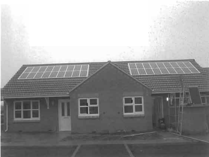
Figure 1 Corncroft development, Nottingham, UK.
