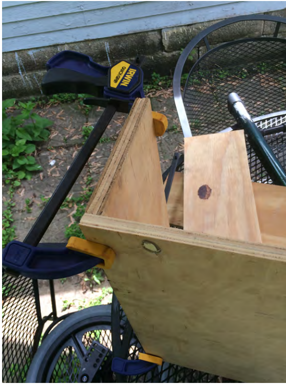
Figure 11-14 Begin making the cargo box out of plywood
