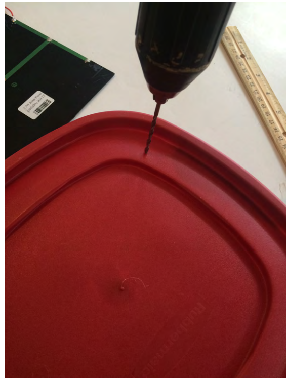
Figure 8-8 Drill holes in the sandwich box with identical spacing as the solar panel's wires
