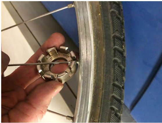
Figure 6-12 Tighten the nipple using your spoke wrench
