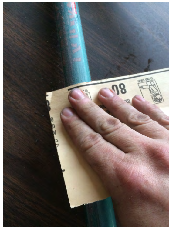
Figure 5-17 Sand the surface of the existing paint job
