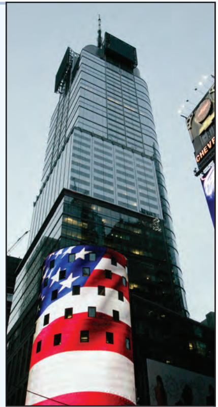
Parts of the south and east faces of the Condé Nast Building in New York City include thin-film solar panels.
