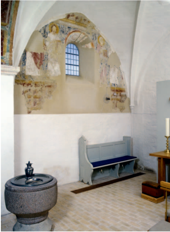
Figure 8.3 The aesthetic enhancement of the Romanesque wall paintings executed in 1989 in Gundsømagle Church was limited to plaster repairs tinted with coloured sand. Photo reproduced with permission from R. Fortuna.
