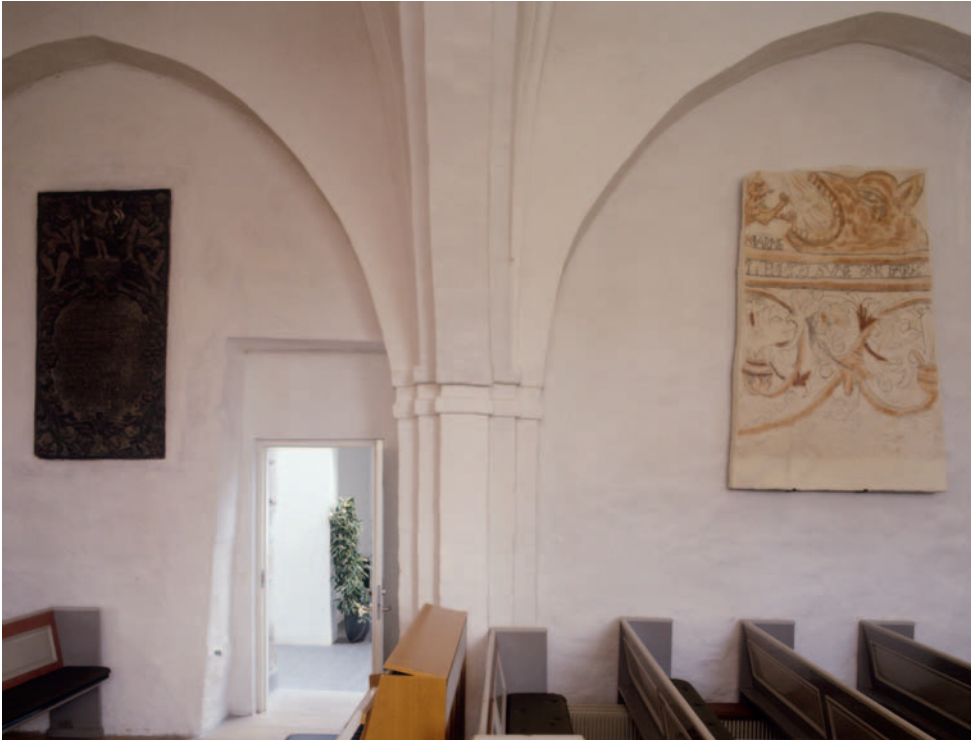
Figure 8.6 The fragment of the Gothic wall painting found in the niche formed by the bricked-in door was detached, transferred to a movable support that replicated the surface configuration, and is now displayed on the wall in Hedensted Church, east of its original location. Photo reproduced with permission from R. Fortuna.
