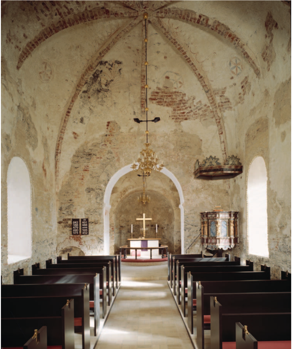
Figure 8.5 Vrigsted Church, view toward east, after renovation in 2001. The concept of the renovation was to expose all the historically significant layers simultaneously, in the condition they were found. Photo reproduced with permission from R. Fortuna.
