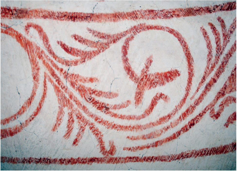
Figure 8.8 Detail of the wall paintings in Vallensbæk Church showing the reconstructed areas intentionally executed with crude brushstrokes in order to achieve the same visual effect as the damaged original paint layer. Photo reproduced with permission from Isabelle Brajer.
