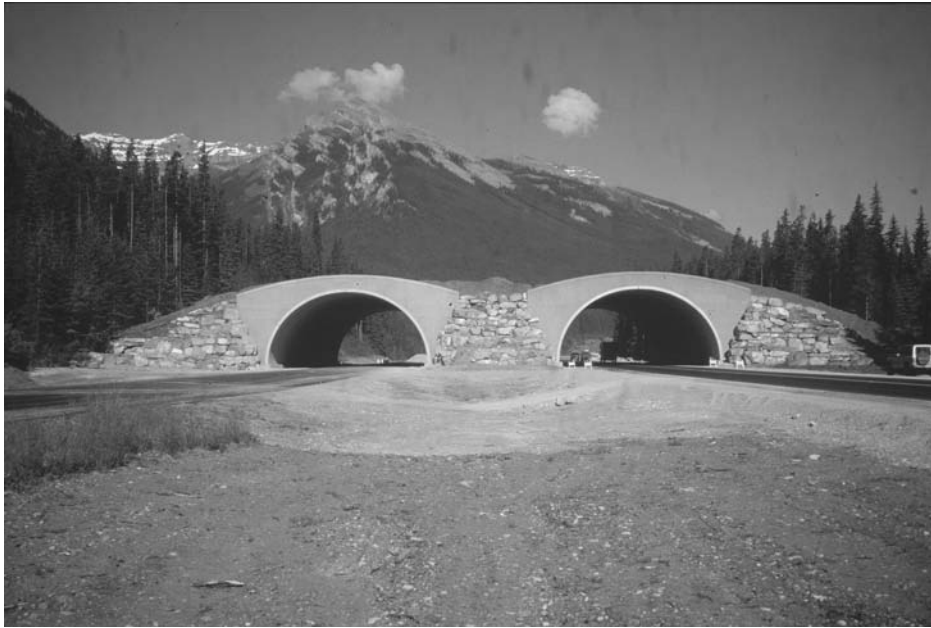
Figure 9.4. An overpass crossing the Trans-Canada Highway in Alberta. This structure allows wolves and other large mammals to safely cross a landscape fragmented by highways. (Photo by Ben Alexander.)
