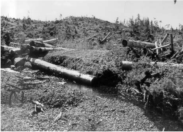
Figure A. A former logging road crossing of a salmon stream in the Copper River delta. Road material is eroding into the streambed behind a leftover bridge stringer log. (Photo by P. Swartzbart.)
