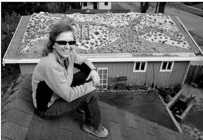
Vivian deZwager shows off the newly planted green roof on her garage. Such roofs help reduce carbon dioxide, as well as heating and cooling costs. Treating the planting as an artistic project may help motivate others to follow suit. (Janet Jensen/MCT/Landov)
