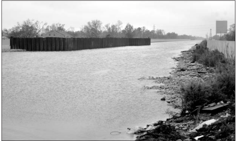
A reinforced section of New Orleans's 17th Street levee, which was breached during the floods associated with Hurricane Katrina. (AP/Wide World Photos)
