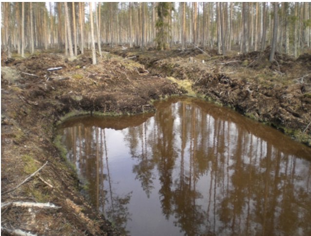
Fig. 17.3 A sedimentation pond constructed to stop soil erosion from a drainage area (Photo: Leena Finér)
