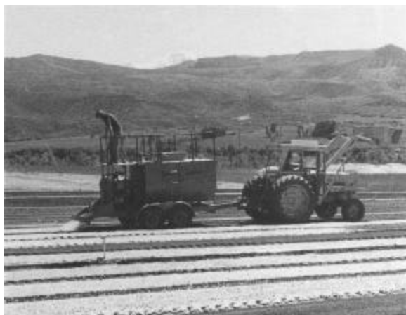
Figure 14. Hydromulcher spraying a mulch-water mixture on prepared beds.
