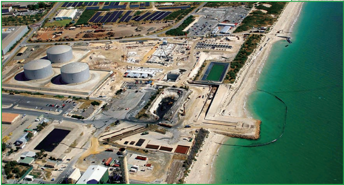
The seawater desalination plant in Perth, Australia, is the largest in the Southern Hemisphere. Desalination is expected to become increasingly critical as a source of safe, clean water. (ABB Engineering)
