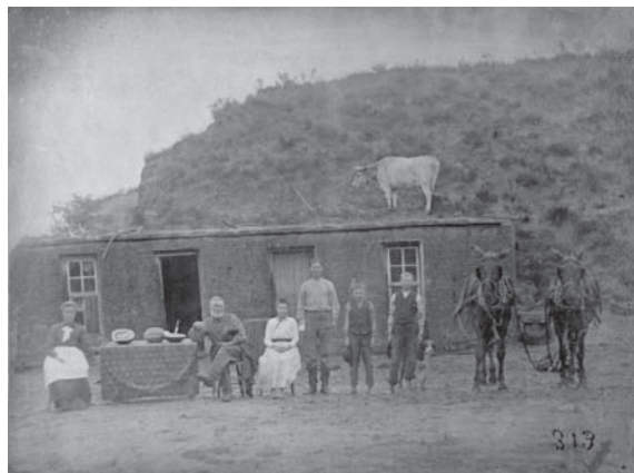
Figure 4-4 Sod house in late 18th century North American prairie. Thousands of such houses dotted the prairies of North America at this time.
