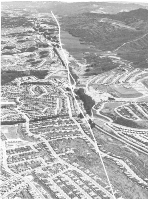
Figure 13.21 Housing tracts constructed within the San Andreas fault zone, San Francisco Peninsula, before the state passed legislation restricting this practice. The white line indicates the approximate fault trace, along which the ground ruptured and slipped about 2 m during the earthquake of 1906. [R. E. Wallace/USGS.]
