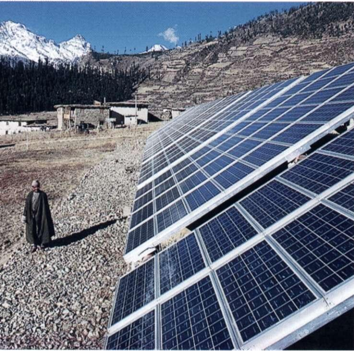
Figure 23.16 Solar cells convert sunlight, a renewable resource, into electric energy at this utility in a remote village in Nepal. [Ned Gillette/Corbis.]
