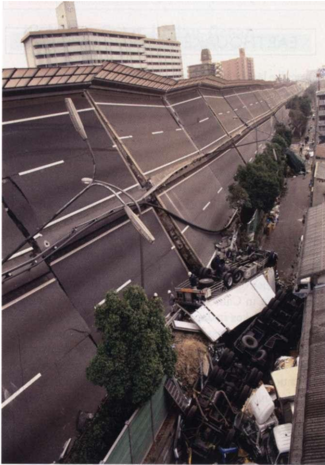
Figure 13.15 This elevated expressway, in Kobe, Japan, was overturned during an earthquake in 1995. [Tom Wagner/Corbis/SABA.]
