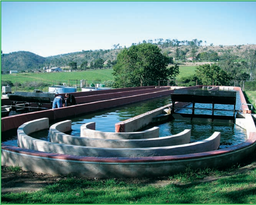
This artificial wetland in South Africa uses algae in a continuous-flow pond to further treat effluent from a municipal sewage treatment plant. ( WIO-Lab Project, United Nations Environment Programme )
