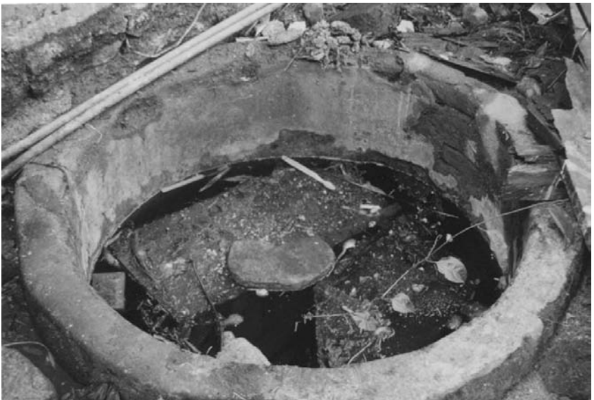
Fig. 5.5. An abandoned drinking water well in the Moratuwa-Ratmalana area polluted by textile industry effluents
