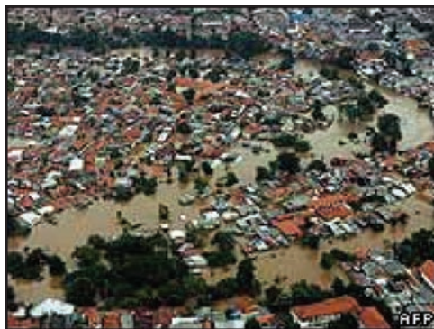
Figure 2.8 Flooded densely populated area of the city at Jakarta, Indonesia, February 2008.
