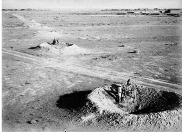
Fig. 8.4 Constructing qanats using reinforcing rings. Note the spoil crater from digging the well. (Source: Ghayour 2000)
