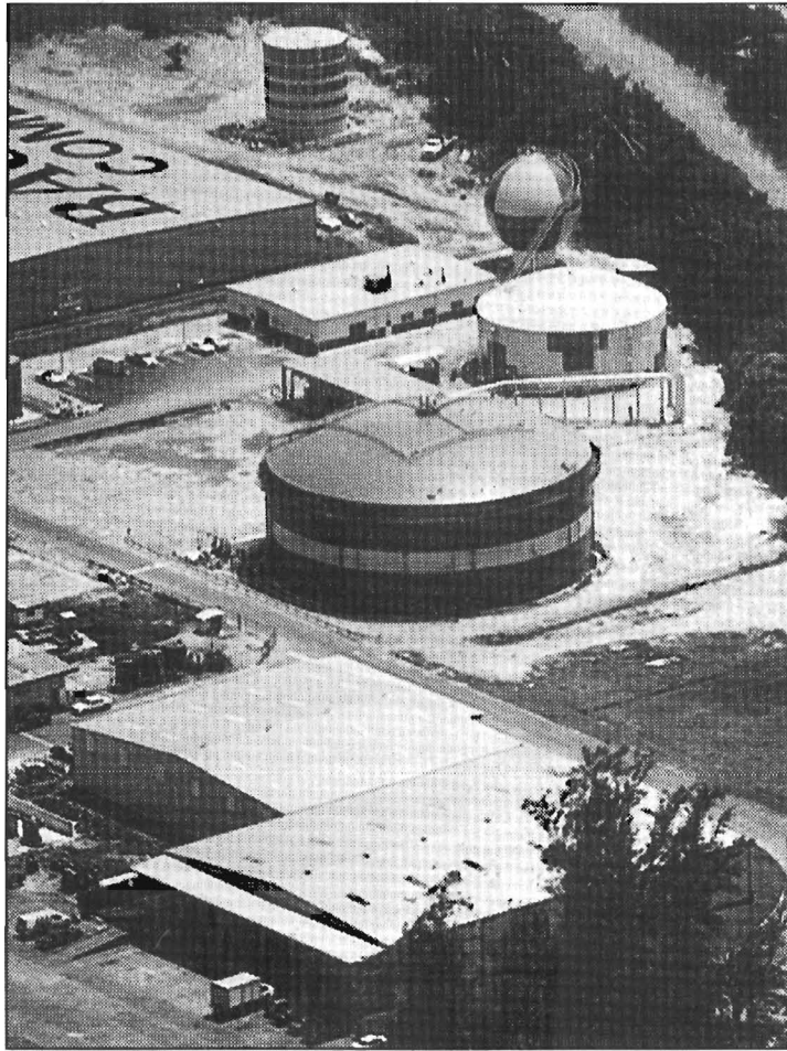
Photo 13.3 Packed-bed anaerobic filter with plastic media used to treat rum wastewater.
