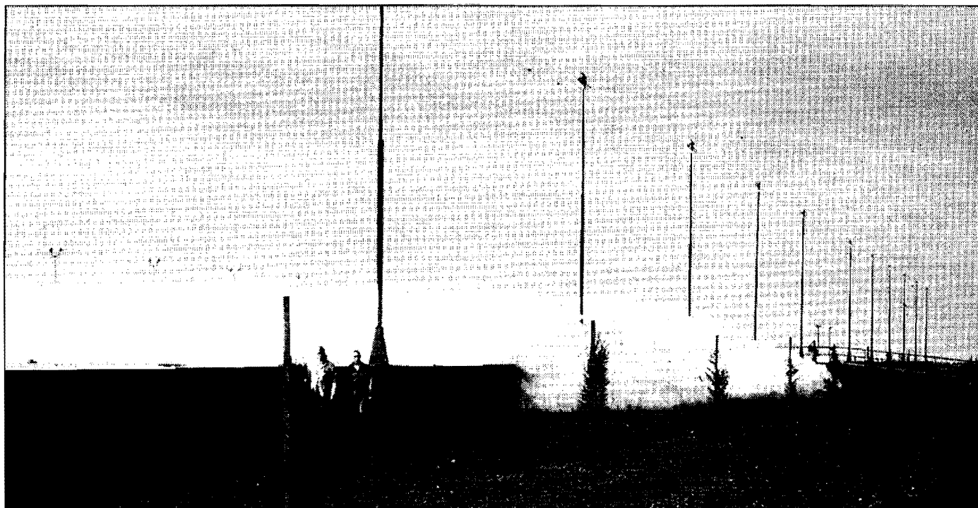
Figure 14.1 Foaming at an activated sludge plant due to ABS detergents in the early 1960s (courtesy of Bruce M. Wyckoff).
