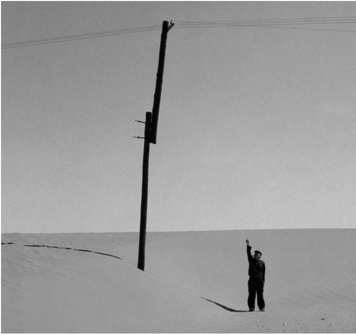
After more sand storms, the accumulating sand is carried to another location, leaving the extended pole far above the lowered land surface. Photo: Lu Tongjing.
