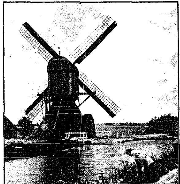
Fig 13. Traditional Windmills. (Upper left) Great Chishill post-mill, Cambridgeshire, oriented by a fantail. (Lower left) Chesterton tower-mill: 19th century photograph of a unique structure, possibly designed by Inigo Jones: oriented by a winch inside the cap. (Below) Dutch 'Waterwipmolen': a drainage post-mill oriented by a capstan wheel. (Top right) 'Tjasker', smallest and simplest type of Dutch drainage mill lifting water by means of an Archimedian screw. (Lower right) A 'paltrok', a uniquely Dutch type, designed for sawing wood. The entire structure rotated on rollers on a brick base. (Far right) The most characteristic Dutch type, a thatched smock-mill oriented from the outside by a capstan wheel and spars attached to the cap.
