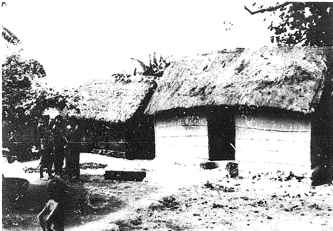
A typical village home with walls made of bamboo sticks and a thatched roof of rice straw
