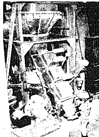
Mini cement plant: a portion of the bottom of the shaft kiln showing the discharge gates and the grate shaft (CRI, Ballabgarh, Haryana)
