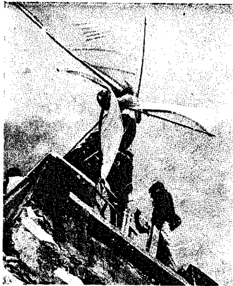
Fig. 6. Deep well windpump built by village artisans, designed by Marcus Sherman.
