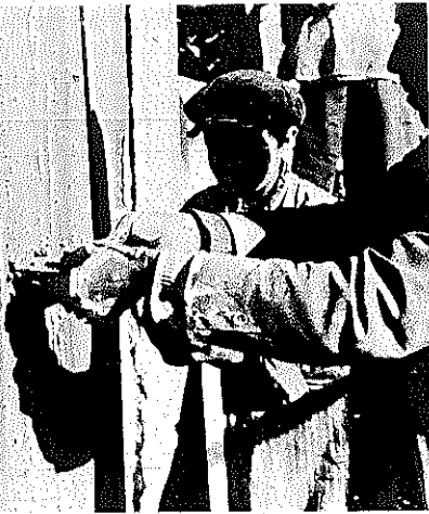
Figure 210 Molding Plaster with a Board
