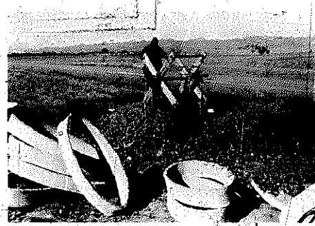
Figure 338 Qanât-Lining Hoops
