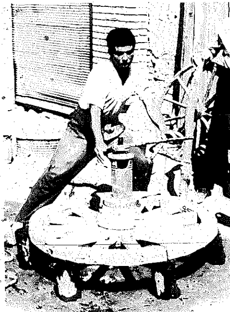
Figure 132 A Wheelwright Bushing a Wheel
