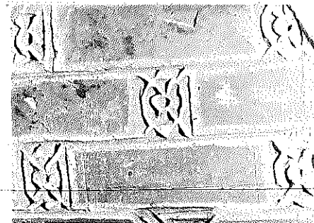
Figure 178 Carved Plugs in Brick Joints at Sultāniyeh
