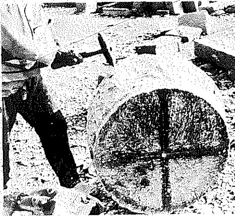
Figure 197 Mason Roughing (Squaring) Column Base
