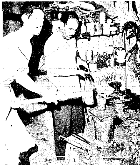
Figure 71 An Anvil Placed on a Wooden Block
