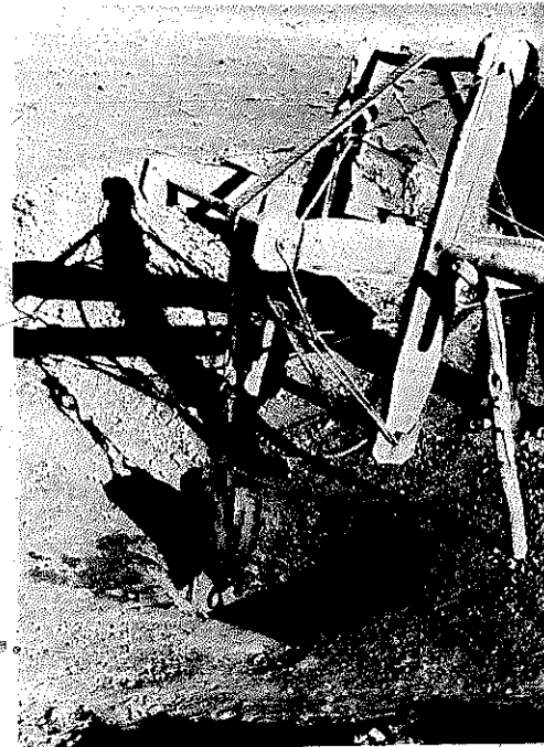
Figure 335 A Winch Bringing the Spoil to the Surface
