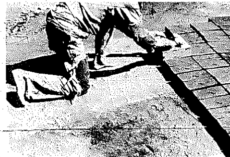
Figure 173 Emptying the Brick Mold
