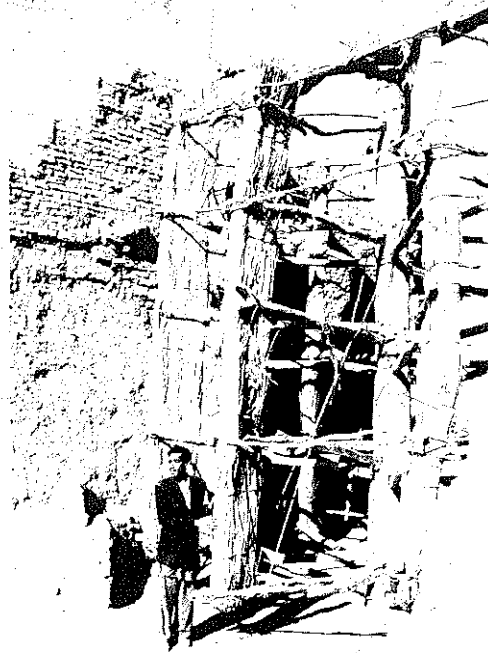
Figure 404 The Wind Wheel of the Sistani Mill
