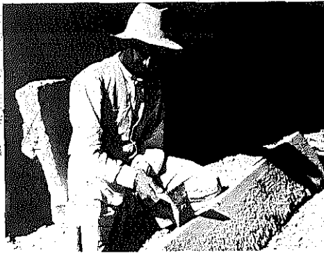
Figure 198 Mason Smoothing Stone with Kernel Hammer
