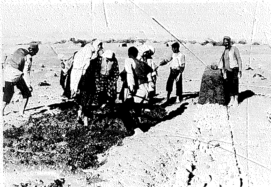
Figure 161 The Building of a Pisé Wall
