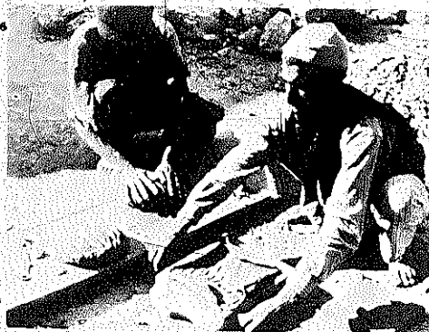
Figure 235 Cutting Away Surplus Clay
