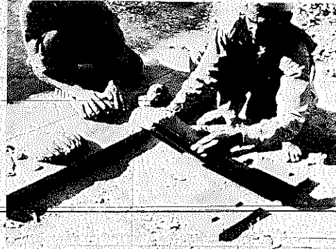
Figure 236 Taking Tile out of the Mold
