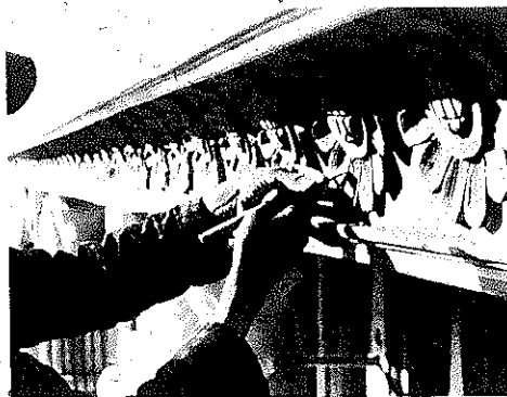
Figure 211 The Carving of Stucco Plaster
