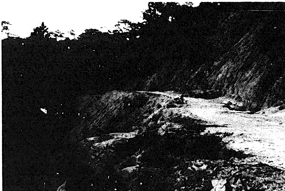
Road construction causing massive soil erosion, Honduras (Stern).
