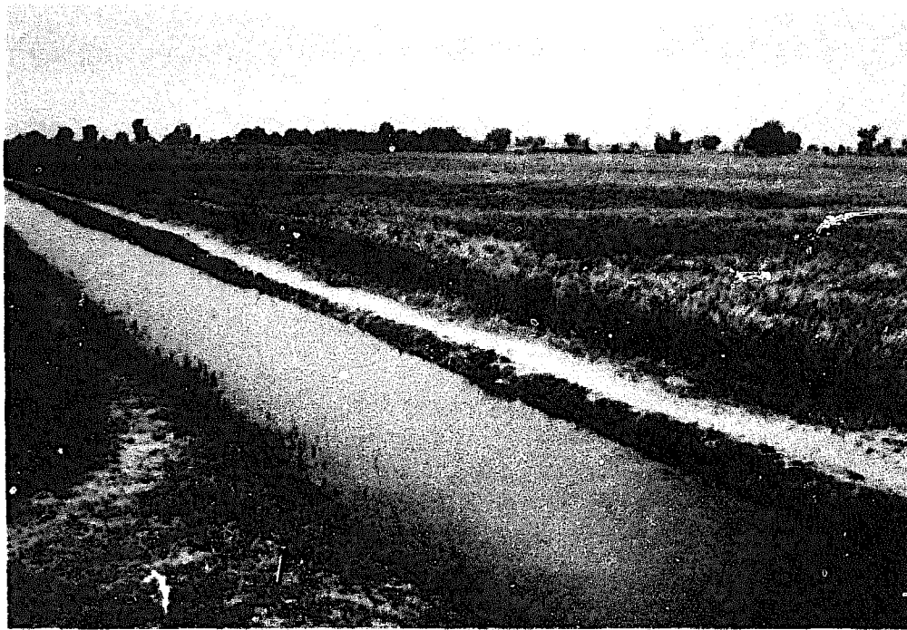
Irrigation supply channel.
