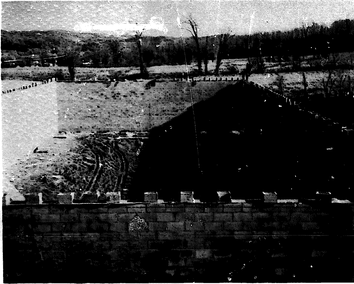
The latest addition at the MacDonald Honey Co. brought the floor area up to a total of 17,000 square feet. Block construction was favored as it is cheaper and can be considered finished inside and out when construction ends.
