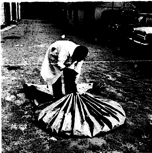
FIGURE 29. The Allgate drier, showing the method of closing in order to give protection against rain and insects.
