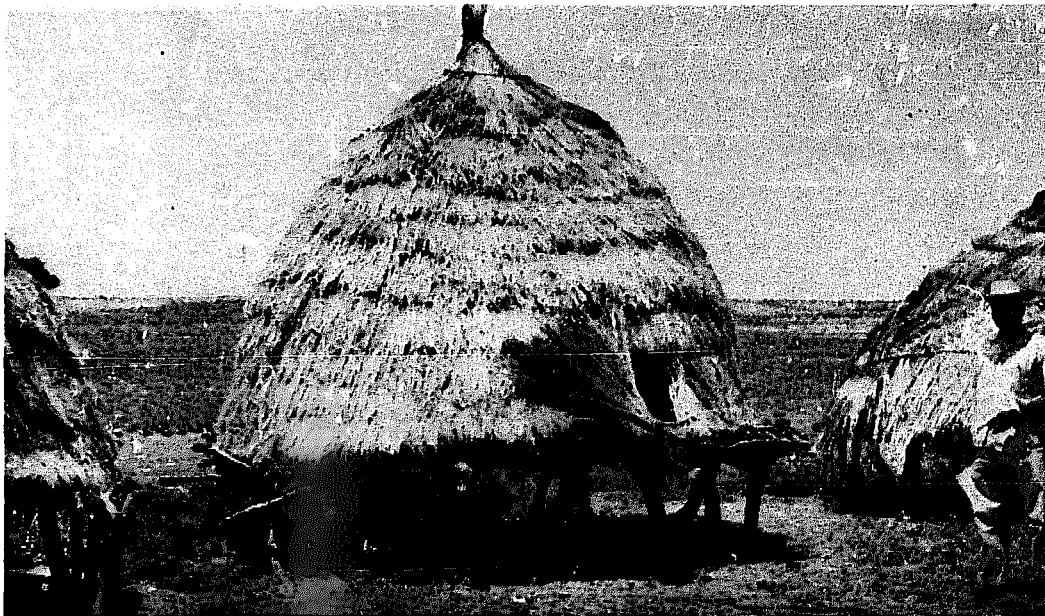
FIGURE 33. Produce on a platform covered by a permanent thatched roof.
