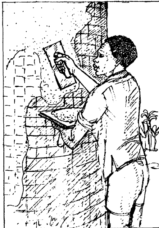
FIGURE 26. Weldmesh type silos. Above, completed silos; right, the hessian/metal matrix onto which cement mortar rendering is being applied.
