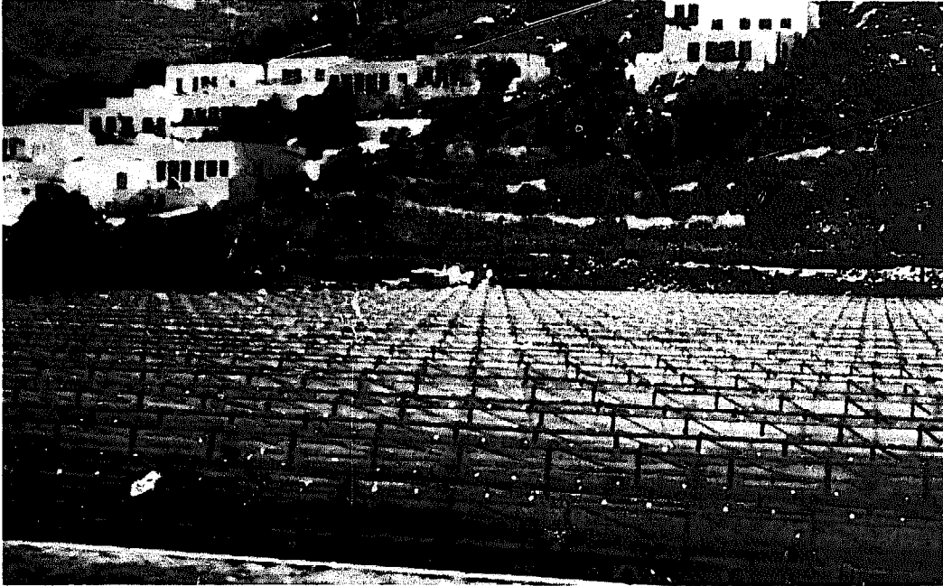
FIGURE 8 Solar still on the island of Patmos, Greece. (Constructed in 1967; total area 95,000 ft 2 [8,826m 2 ])
