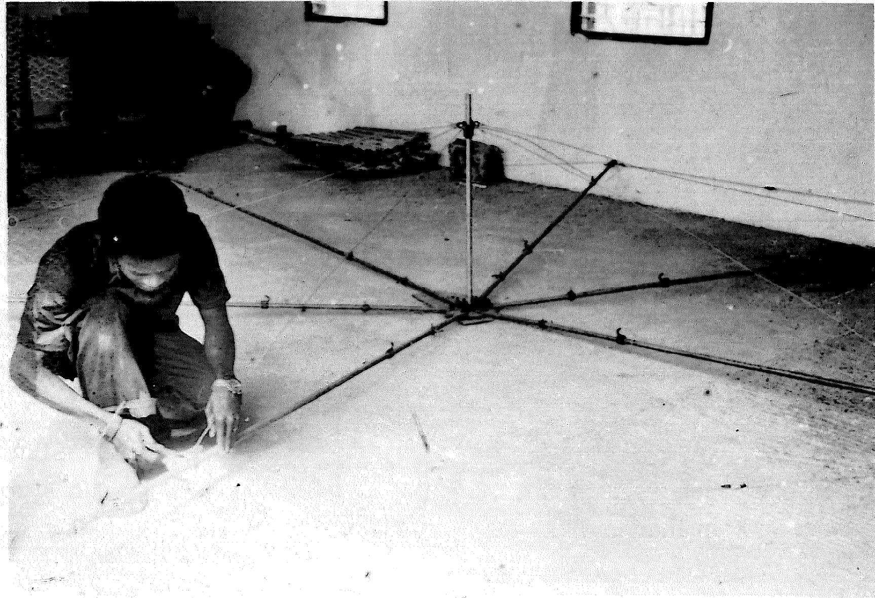
Assembly of wind wheel.
