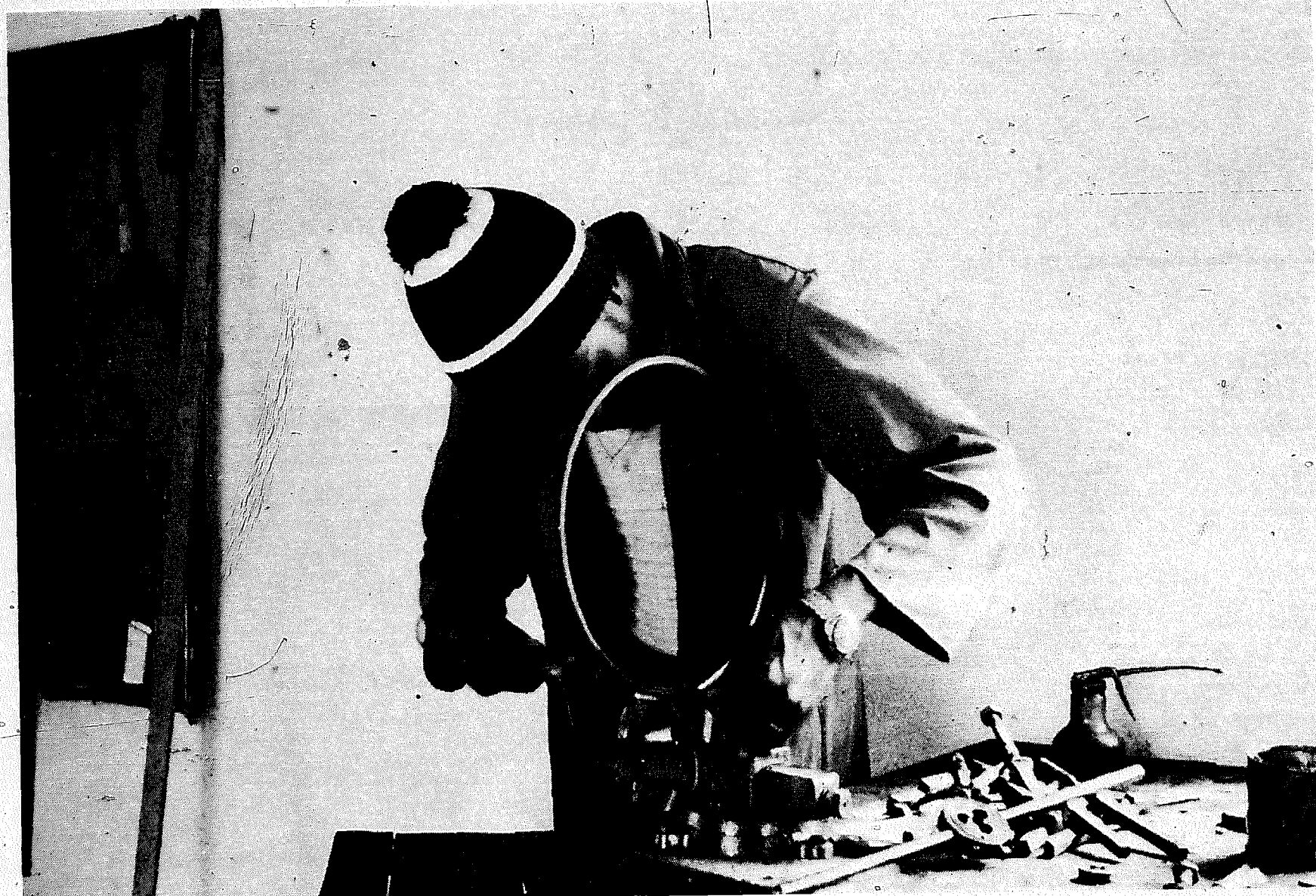
Making a turntable bearing track.
