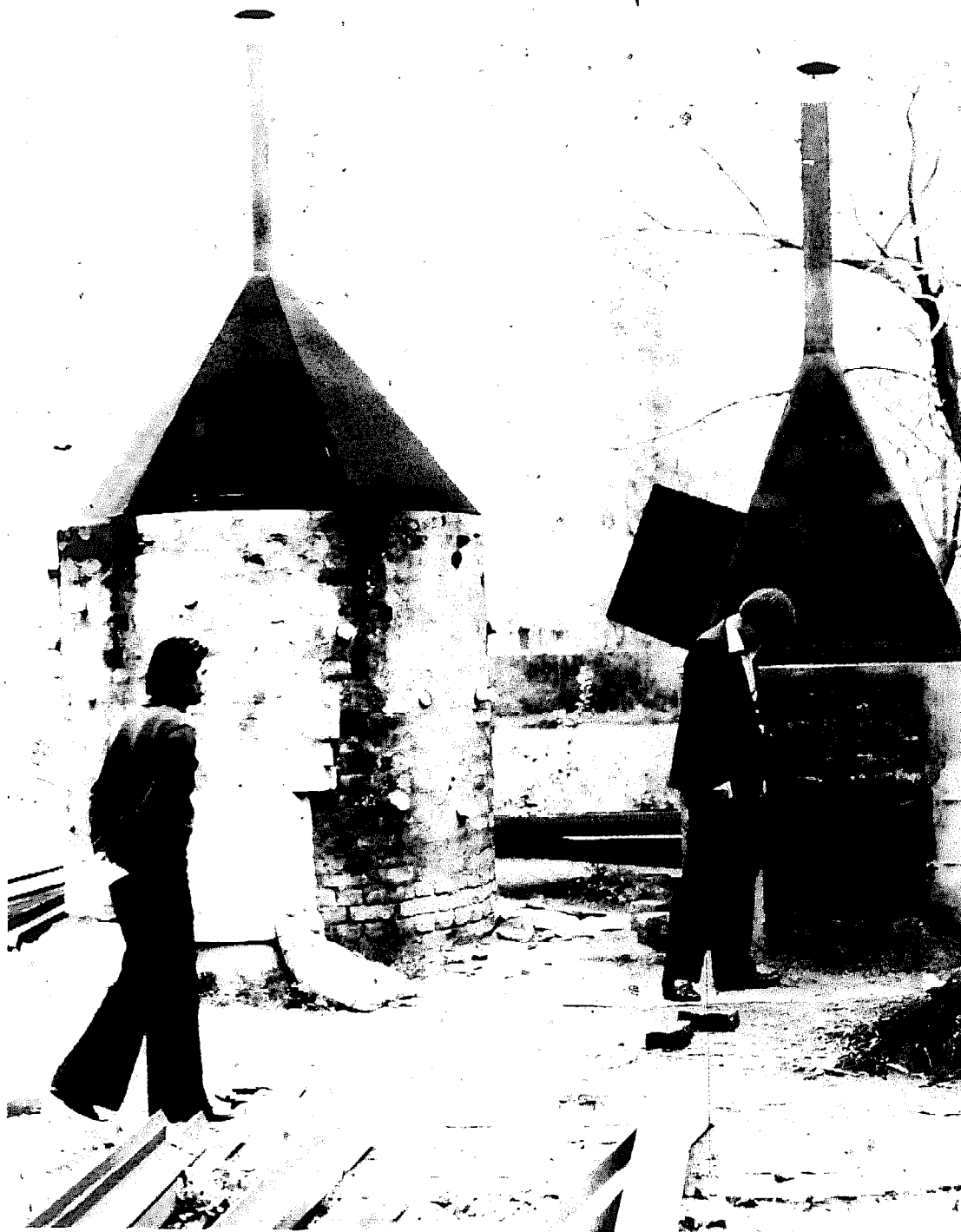
Figure 2. CRI small experimental incinerators at Ballabgah. Left - unsuccessful design. Right - successful design. Dr. S.C. Ahluwalia (CRI). Prof. D.J. Cook (Univ. NSW)
