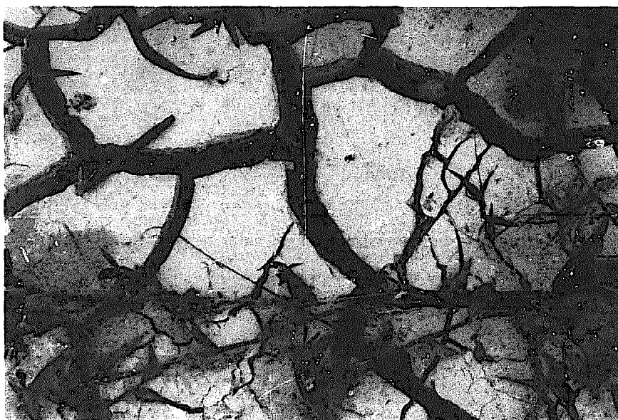
Figure II.7 Shrinkage cracks in clay pit bottom
