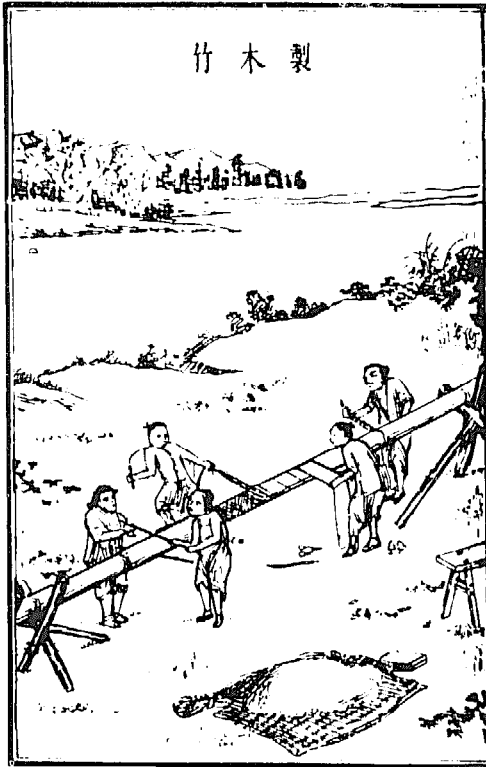
joining bamboo pipes in Szechuan, 1637.
