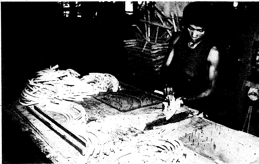
Figure 37. Adjusting moulded components to achieve correct bend. (Note template)
