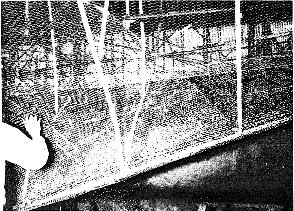
Figure 4-7. Second layer of inner mesh being laid. Note first layer laid fore and aft and the amount of overlap to each strake of mesh
