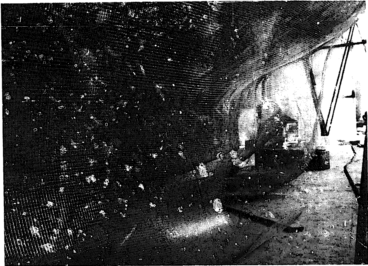
Figure 4-13. First layers of square welded outer mesh hung in position from sheer. Tying commences at top of sheer and works progressively down the hull to underside of keel
