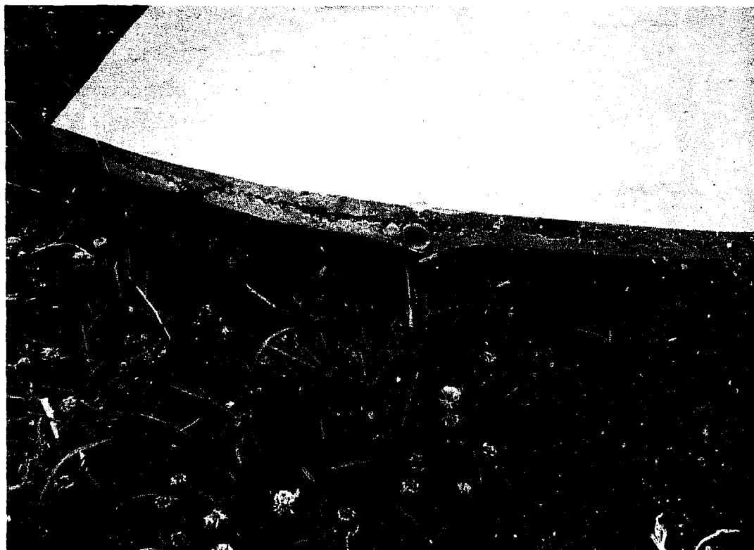
Figure 6. Lamination in the skin of the hull caused by air trapped during the plastering process
