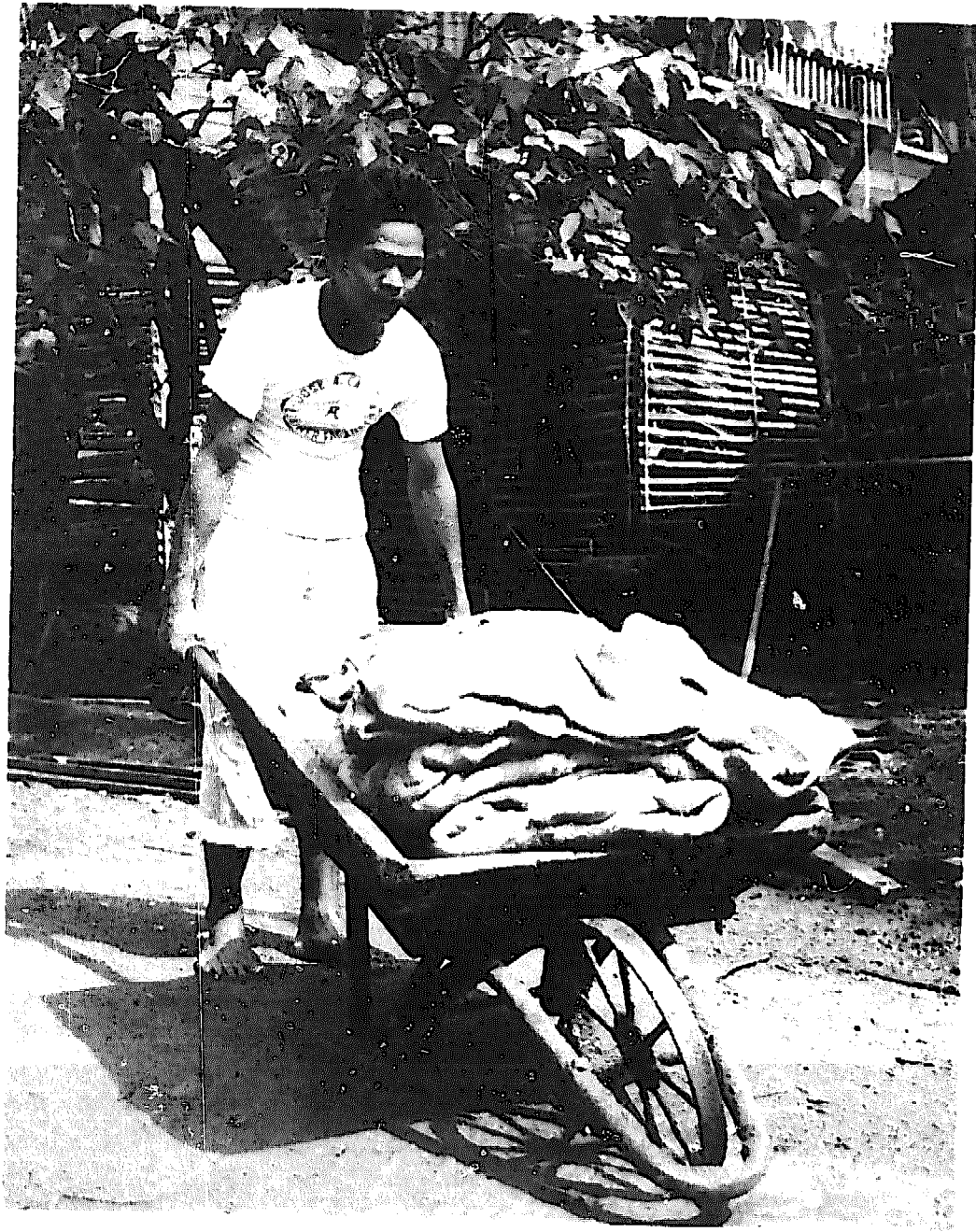
A western wheelbarrow with steel frame and wheel, and a wooden body. (UNA)
