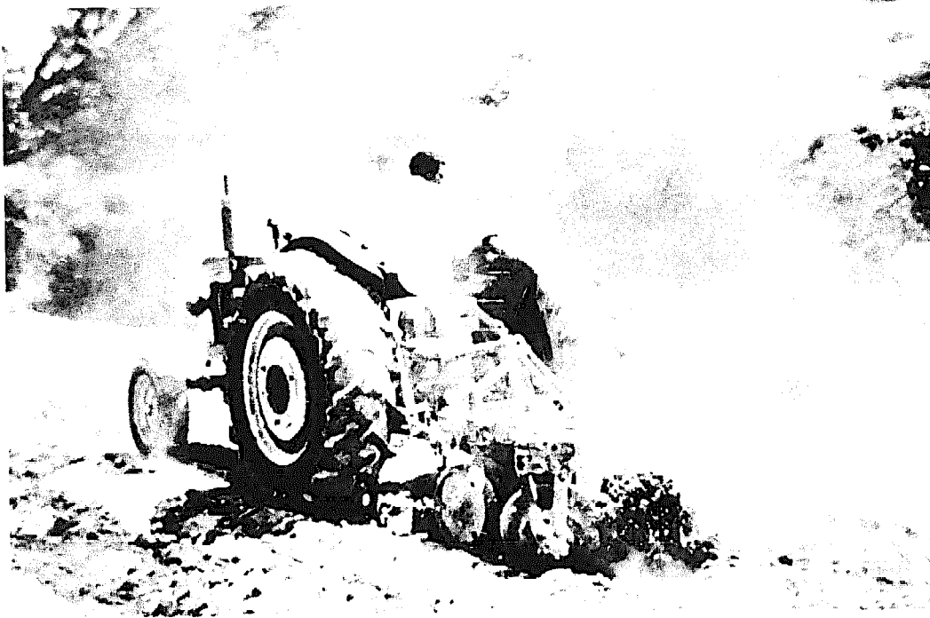
Figure 6. Lime stabilisation: a rotary plough raises a cloud of lime dust
