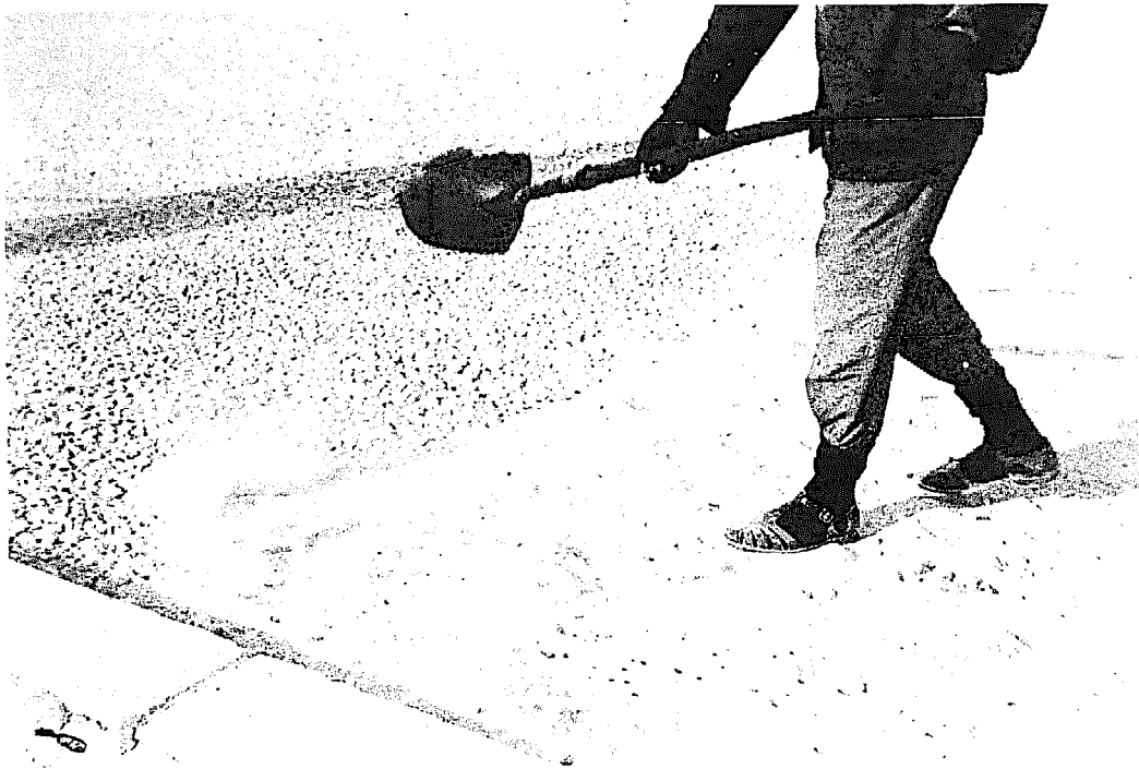
Figure 3. Spreading fine aggregate for dry-bound macadam
