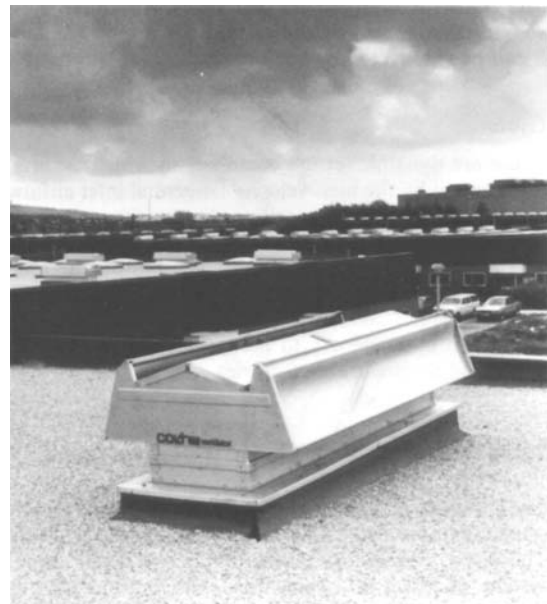
Figure 28.9 Weathered roof ventilator
