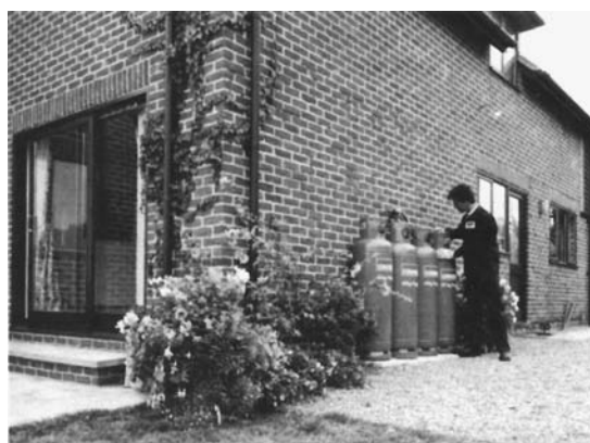
Figure 20.10 A 2 x 2 LPG cylinder pack supply domestic premises. (Courtesy of the Calor Group Plc)
