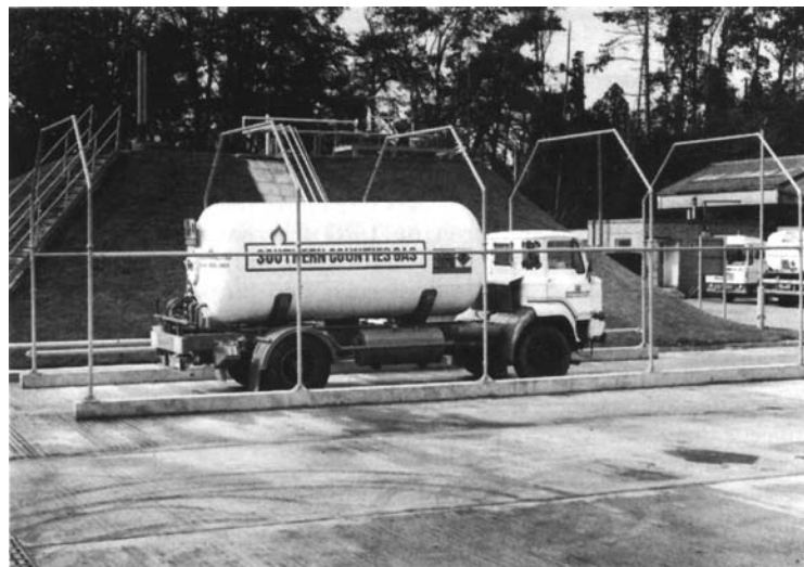
Figure 20.8 Mounded LPG storage. (Courtesy of Southern Counties Gas)
