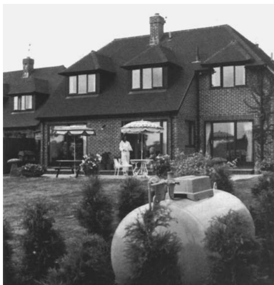
Figure 20.5 LPG storage vessel for a domestic installation. (Courtesy of the Calor Group Plc)
