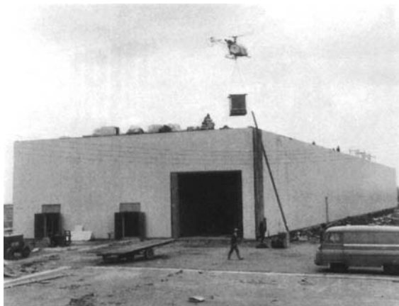
Figure 34.8 Cranes can be eliminated!
