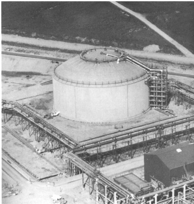
Figure 20.3 Refrigerated LPG storage at 'Flotta'. (Courtesy of the Motherwell Bridge Group)
