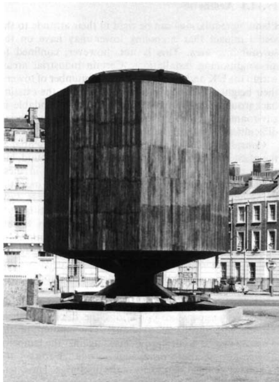
Figure 34.7 Design requested by architect – low plume, no splash (note catchment tray), clear of office block
