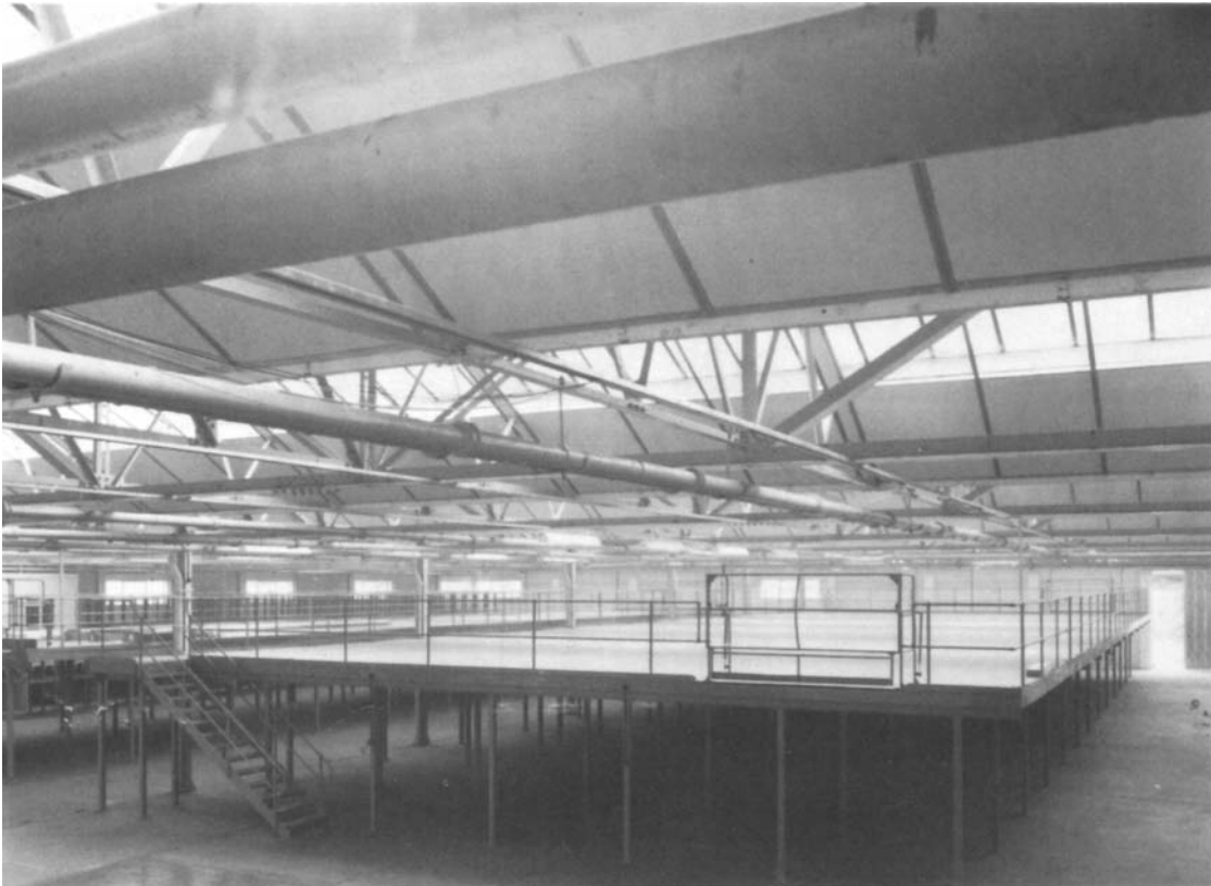
Figure 6.11 A typical modular mezzanine floor (courtesy of The Welconstruct Co. Ltd)
