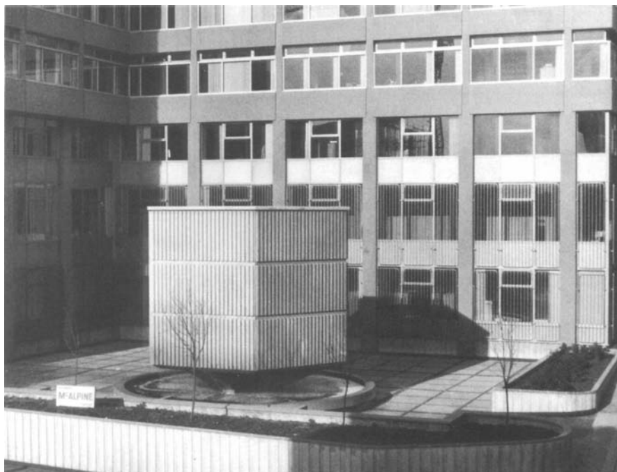
Figure 34.4 Architect-designed tower (note water pattern in basin). Chemicals in carry-over affect the office windows
