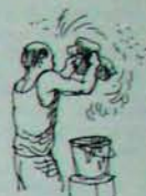
BAGGING THE WALL
