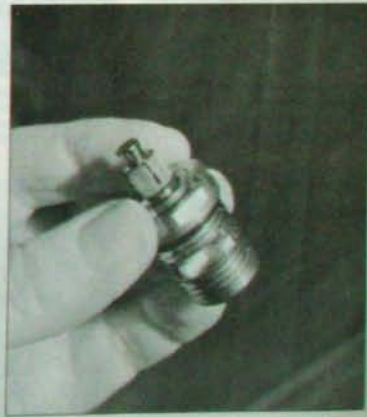
6 Make sure that the new cartridge is correctly 'handed' and screw it into the tap body. Re-assemble the components of the handle in the reverse order of dismantling. Re-secure the water supply, and when it is running freely, close the tap.
