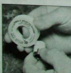
PTFE tape is useful for sealing threaded joints. It should be wound several times around the thread.
