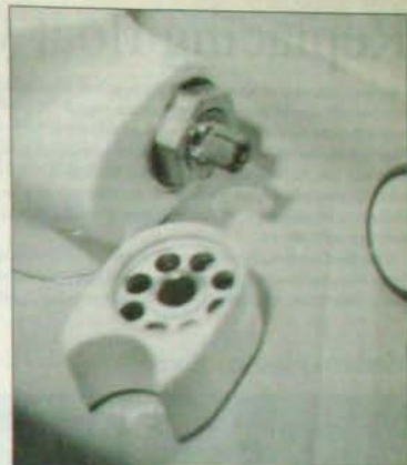
4 Pull the handle off the splined shaft to reveal the top of the cartridge. In some cases, the handle may be fitted to a splined plastic insert which, in turn, is pushed onto the end of the cartridge spindle.
