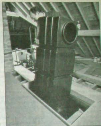
Above A modern loft hatch may not be large enough to permit the passage of a cistern of conventional shape. For such situations, longer versions of small cross-section are available (All illustrations courtesy T & D Trident)
