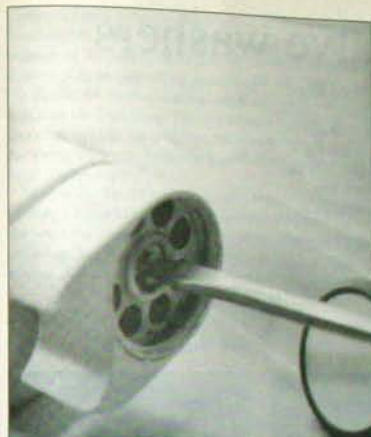
3 With the insert removed from the end of the handle, the handle fixing screw will be revealed. Slacken the screw to free the handle. Some handles will be held in place by a large metal disc as well as the screw.
