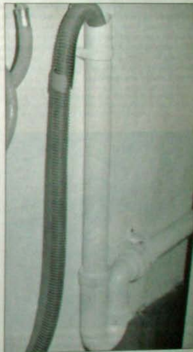
Waste water from the machine may be piped into the waste system of the sink unit via a special adaptor or, as here, into a separate waste pipe with trap. The pipe itself should be laid to a minimum fall of 1:40 to the soil stack or drain.
