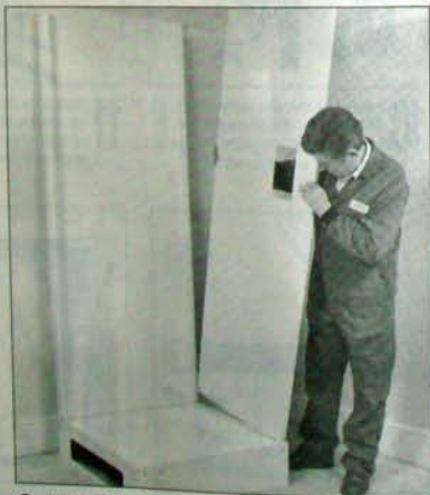
2 Stand the tray close to the final position of the cubicle, but leaving room to work around it. After identifying the back and side panels, they can be loosely secured to the tray with the screws provided.
