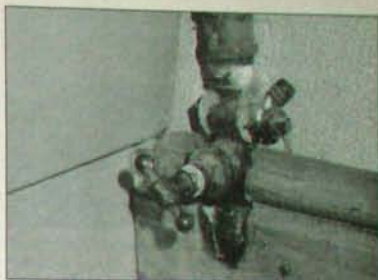
Make sure you know the location of your stoptap; turn the handle regularly to ensure free movement.
