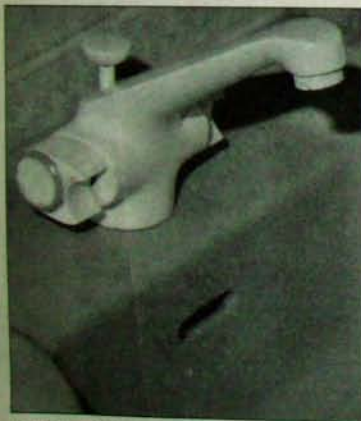
1 This monobloc basin mixer with pop-up waste is fitted with quarter-turn ceramic disc cartridges instead of conventional washers. The cartridges are 'handed' to allow operation in the correct direction depending on where they are fitted.
