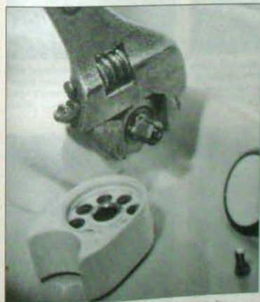
5 Use an adjustable spanner to unscrew the ceramic disc cartridge from the body of the tap. Take care not to slip with the spanner, as its handle may damage adjacent tiling or the top of the washbasin.
