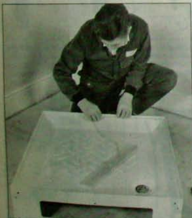
1 After unpacking and checking the components of the cubicle, the waste is fitted to the tray and a sealing strip applied to the top of the tray. A combined waste and trap is available that clears the floor. (All photographs courtesy Leisure)
