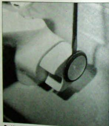
2 After shutting off the water to the appropriate side of the tap and letting the pipe drain, remove the colour-coded insert from the tap top, using a thin screwdriver. Take great care not to damage the handle of the tap or the insert itself.
