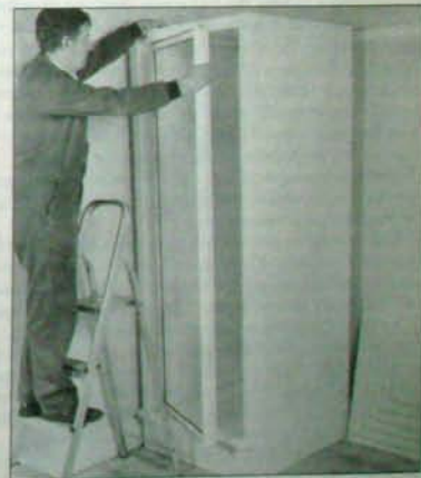
6 After moving the cubicle to its final position, the door can be fitted on its pivot pin (or a curtain hung). All that remains is to connect the waste pipe to the drain (or a pump unit), and fit the required shower unit with necessary pipework.
