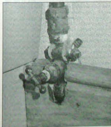
A stoptap should be fitted to the rising main, close to the point at which it enters the property. This will allow the supply to the whole plumbing system to be shut off.
