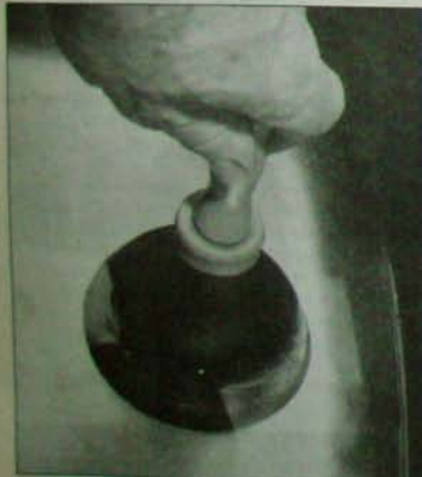
If a sink, basin, bath or shower waste becomes blocked, it can often be cleared with the aid of a plunger.
