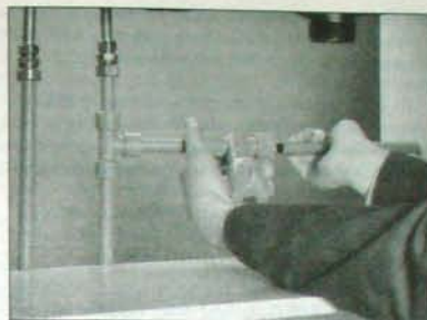
The push-fit fittings used with Hep20 polybutylene pipe make installation quick and simple.
