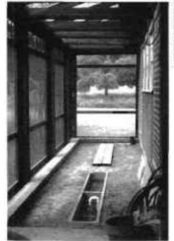
Box troughs water a greywater greenhouse in Maryland.
