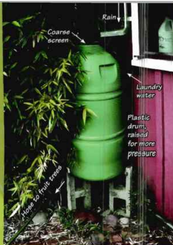
Simple Laundry Drum with Rainwater Harvesting
