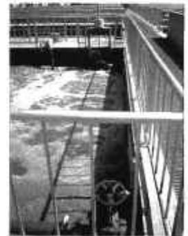
An activated sludge sewage treatment plant dumps greywater in the ocean after energy- and chemical-intensive treatment.
