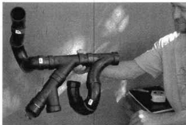
Greywater plumbing subassembled (no glue).
