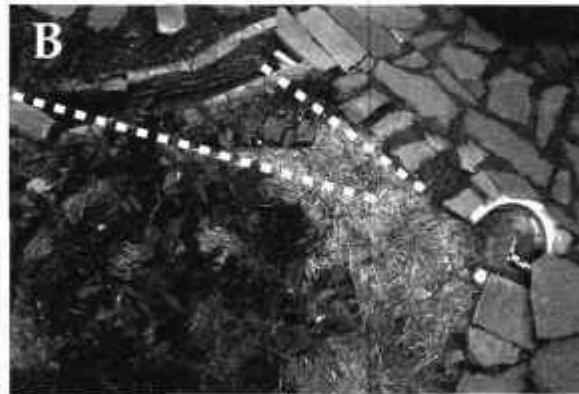
Pipe locations in Huehuetortuga landscape. Positions and orientations of photos A–C are noted on plan above. Path of pipes is shown on photos with dashed lines. It is best to take pictures of pipes before and after they are covered.
