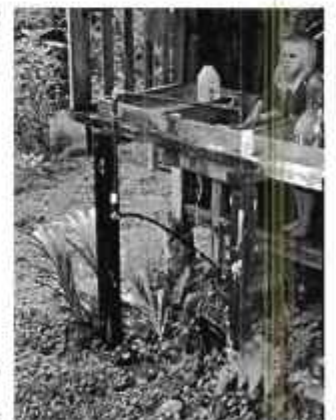
Drain Out Back in Costa Rican rain forest. The water rains into the mini-jungle below, which absorbs and treats it. There isn't even a drainpipe. This system has worked for decades without intervention or problems.
