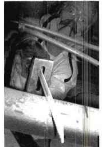
Cutting the old iron pipe with a sawsall.
