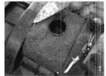
Photo taken by holding the camera down inside the access. Note the bamboo feeder roots coming up through the earth floor.
