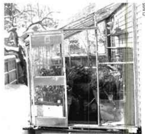
A snowbound greywater greenhouse in Massachusetts, filled with fresh veggies.
