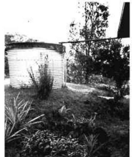
Rainwater harvesting provides all domestic water by gravity for a house near Hilo, HI.
