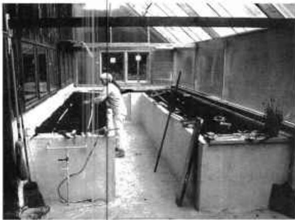
Greenhouse with Clivus Infiltration beds in Massachusetts.
