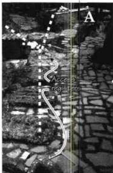
Pipe locations in Huehuetortuga landscape. Positions and orientations of photos A–C are noted on plan above. Path of pipes is shown on photos with dashed lines. It is best to take pictures of pipes before and after they are covered.
