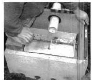
Leveling a dipper: Stand on it and wiggle it down into the concrete while checking levels in both directions.
