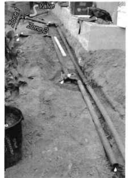
Glued pipes ready for support/burial.
