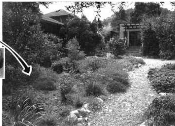
Under these fruit trees are inverted 5 gal pot outlet chambers in large, deep basins. Basins are filled completely with wood chips. The system is completely invisible in the landscape, yet easily serviced by pulling mulch back.
