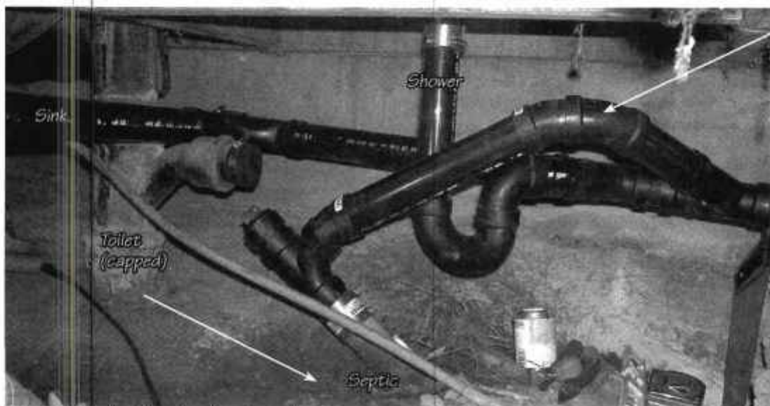
Greywater collection plumbing installed.
