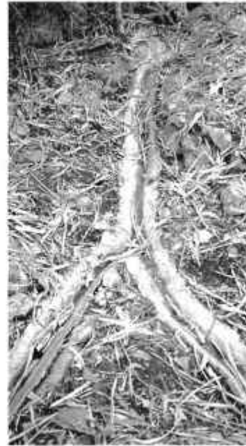
Branched Drain ancestor. A cement channel distributes greywater on a steep, seasonally dry slope in Cuernavaca, Mexico. This system distributes greywater more widely than if it was just dumped on the ground. However, due to imprecisely formed splits, numerous cracks, and blocking from roots and leaves, it is not as predictable as a Branched Drain network. Shaping the splits precisely with a form would help.
