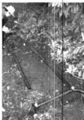
Assembling pipe inside the trenches without glue, and checking levels.
