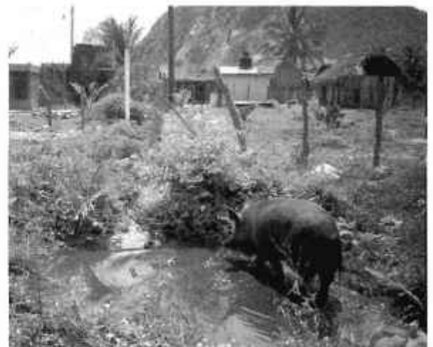
Washwater from a home that feeds a black puddle like this can be rerouted into irrigation furrows (next page), which water and feed about 20 fruit trees. Because the water is spread over a wide area, it never stays on the surface long, so it doesn't stink or breed vermin.
