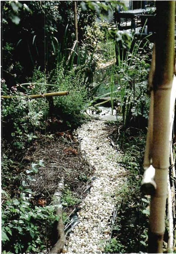
FIGURE C1.8. This plastic-lined, gravel-filled trench directs overflow from the upper garden pond to the lower one. It also collects overland runoff from the upper garden. Notice the vertical piece of bamboo in back; this carries roof runoff from the house into the lower pond. These catchment systems reduce the need to manually fill the pond, while also maintaining habitat for beneficial organisms that use the pond, such as frogs and dragonflies. These reduce pest populations in the garden. This picture was taken about 20 feet (6 m) north of figure C1.4, looking in the same compass bearing. Notice the difference in light conditions. Photo by Dave Jacke.
