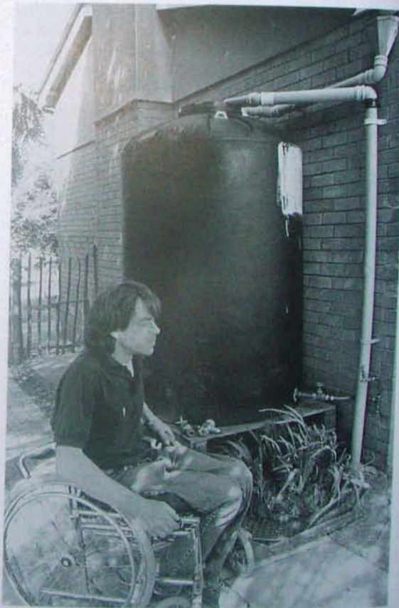
Plate 4.1 Simon Phelps beside his rainwater harvesting system. Note that the tank is raised off the ground so that all the water in it can be used by gravity. (Steve Easton)
