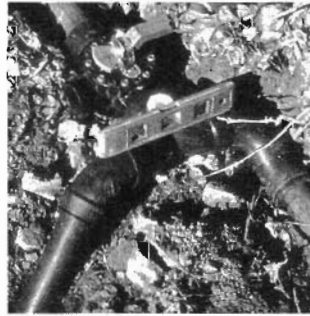
Subassembly is then glued into the system as a unit.
