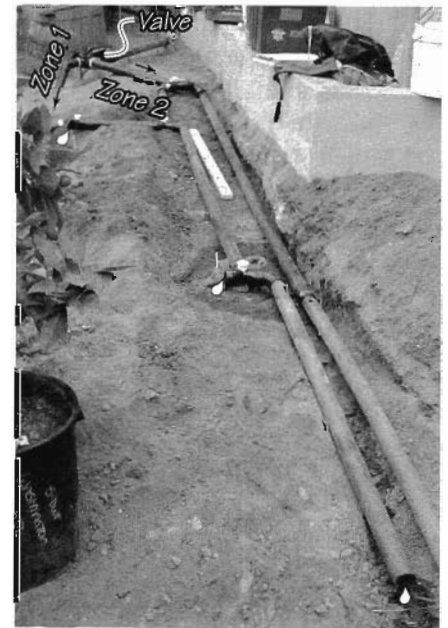
Glued pipes ready for support/burial.
