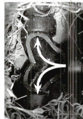
Cutaway view of a double ell, a flow-splitting fitting that is largely self-cleaning with no filtration. This one is part of the first known Branched Drain network. I valiantly tried to clog it with pure kitchen sink water—took the sink strainer out and pushed bowls of soggy granola and pot scrapings down the pipe for half a year. The p-trap clogged every other day, but the Branched Drain network never did.
