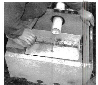
Leveling a dipper: Stand on it and wiggle it down into the concrete while checking levels in both directions.
