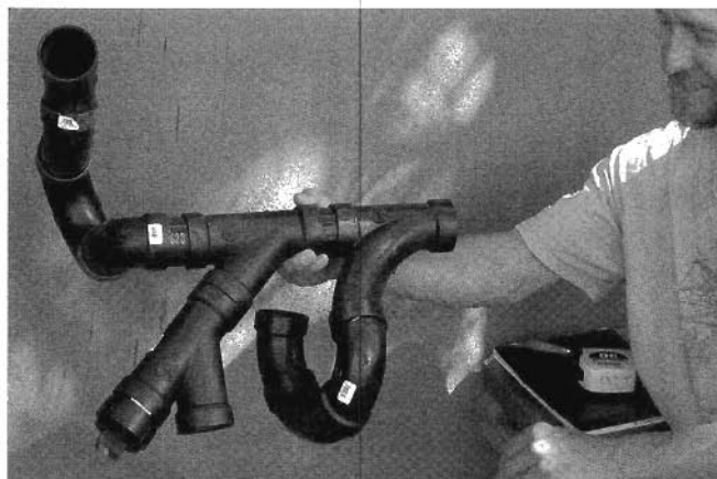
Greywater plumbing subassembled (no glue).
