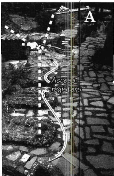
Pipe locations in Huehuetortuga landscape. Positions and orientations of photos A–C are noted on plan above. Path of pipes is shown on photos with dashed lines. It is best to take pictures of pipes before and after they are covered.
