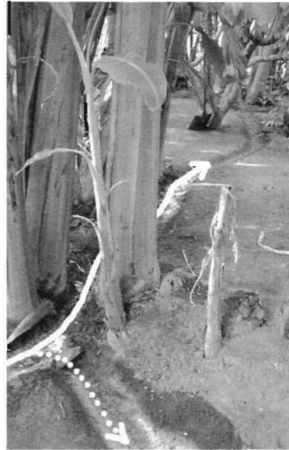
Simplest possible diverter valve: A coconut shell (rock, chunk of wood, dirt clod...whatever) is shifted by foot from blocking one greywater furrow to another.
