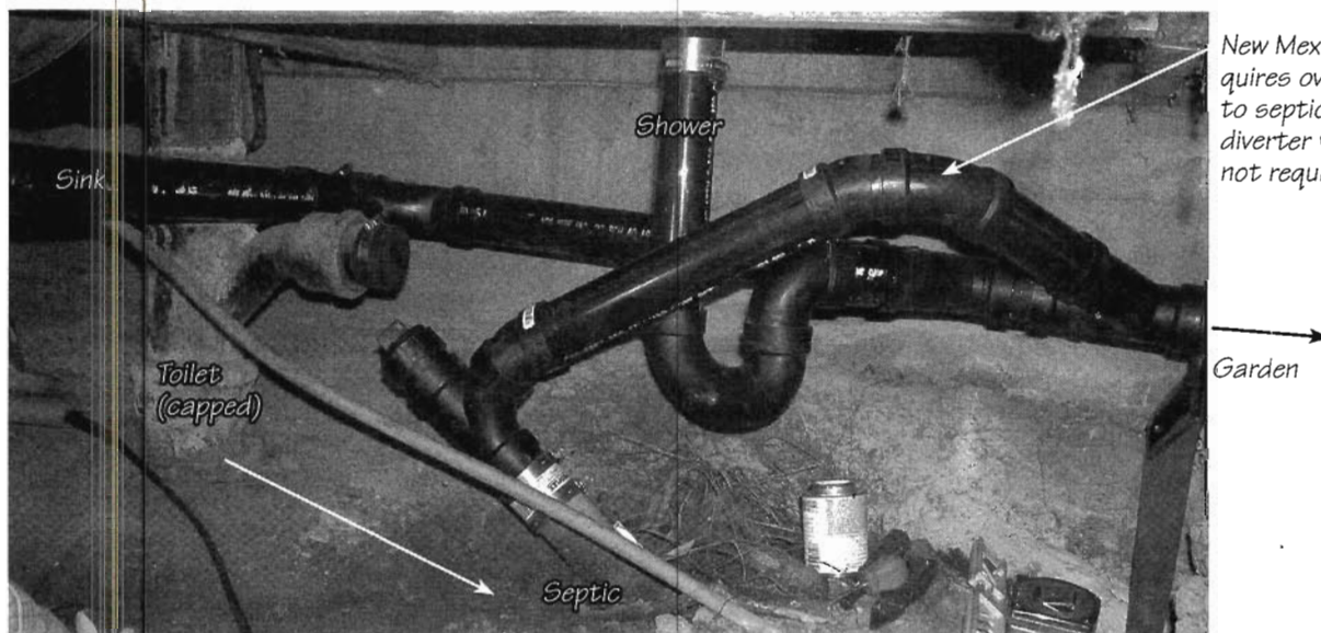
Greywater collection plumbing installed.
