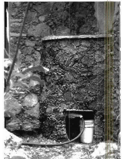
Multi-Mode Greywater Tank with enough fall to fill a bucket from a valve at the bottom. A quarter-cylinder shape, this tank fits nicely in an inside corner of the house. It holds 50 gal (190 L) and is made of ferrocement faced with stone. The floor slopes strongly toward the outlet, so it drains completely of water and is self-cleaning of solids.
