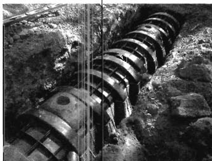
Finished access lids, one per infiltrator. They will have pavers over them on the surface to mark their location.
