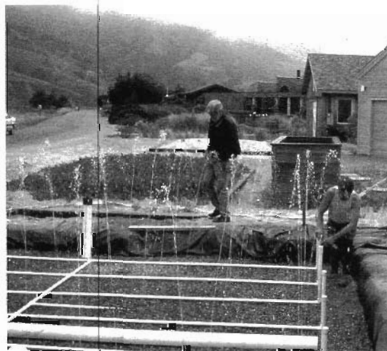
Orenco sand filter system being pressure tested in Stinson Beach, CA. The pipes will be covered with sand and plants. These houses are on a narrow sandbar with ocean on one side and an estuary on the other. As part of one of the most stringent monitoring programs in the country, Stinson Beach inspects all on-site wastewater treatment systems annually.
