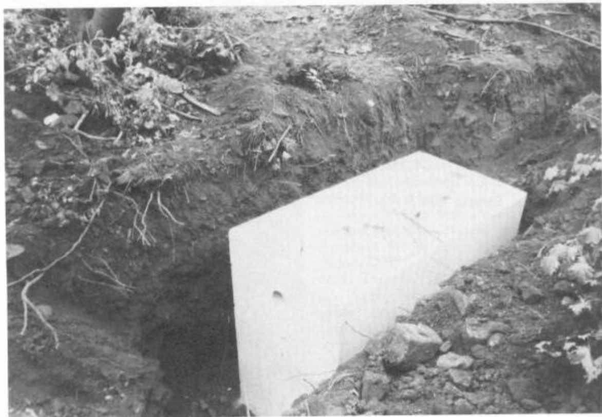
Fig. 6-7. Concrete septic tank in place.
