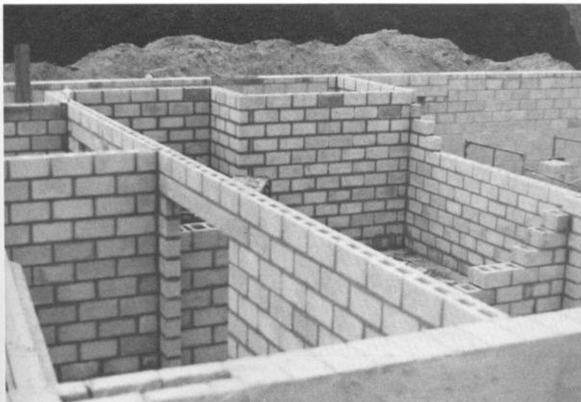
Fig. 8-5. Final stage of blocklaying.
