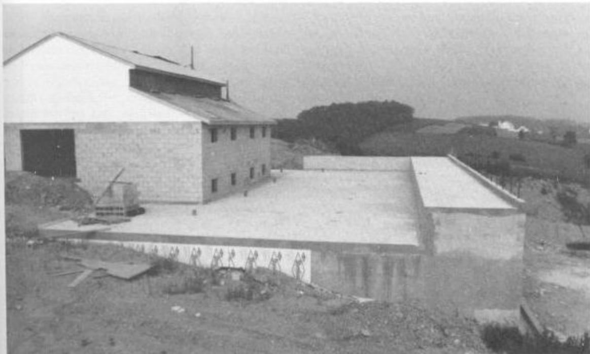
Fig. 10-13. One last view of this earth-sheltered home.
