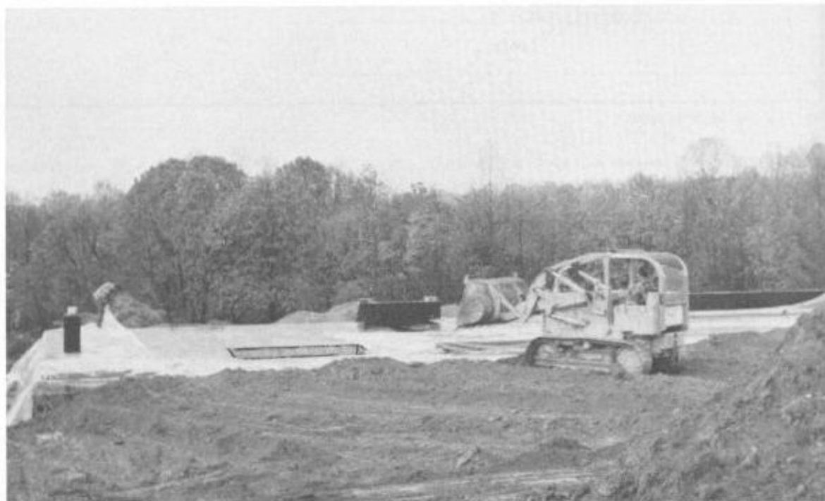
Fig. 11-3. Begin to back fill carefully while watching for large rocks.
