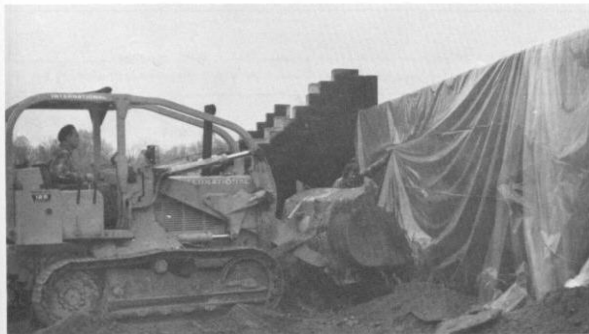
Fig. 13-2. Polyethylene sheets are difficult to keep smooth.
