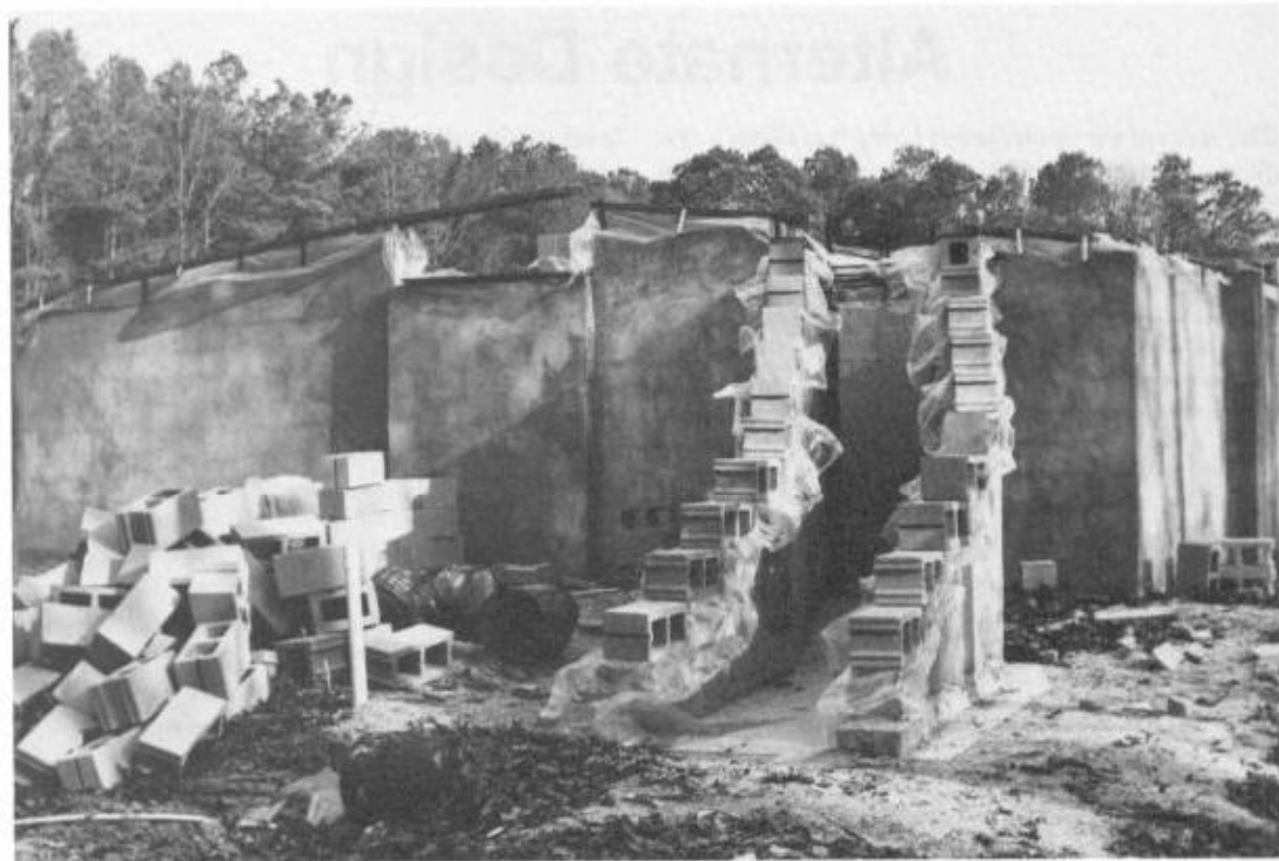
Fig. 10-2. Early stages of blocklaying for this typical home.
