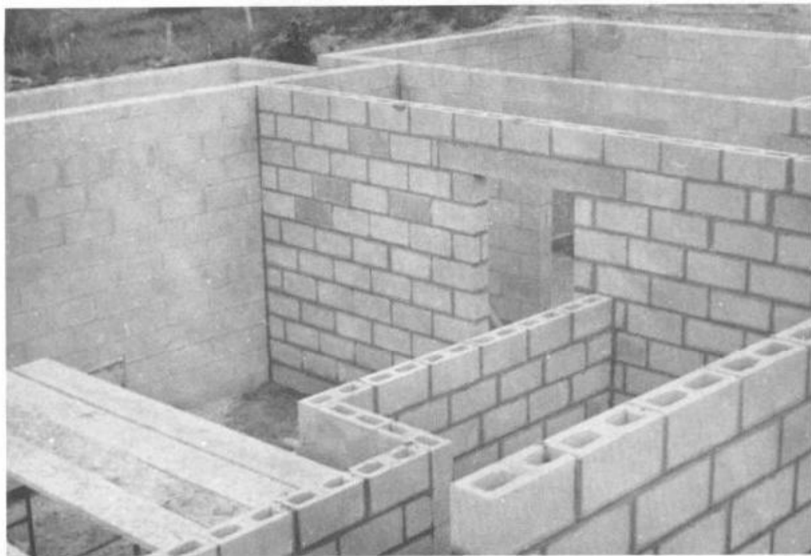
Fig. 8-4. Mid stages of blocklaying.
