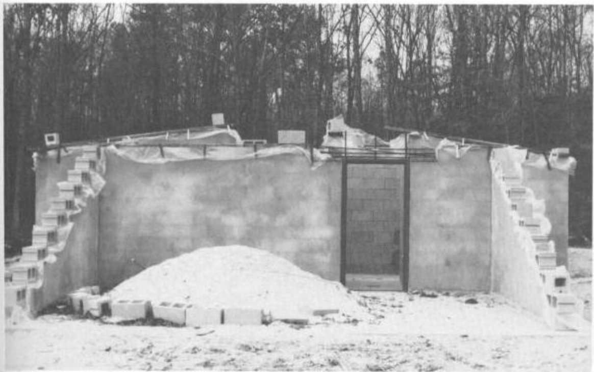
Fig. 10-8. Front view of block construction.
