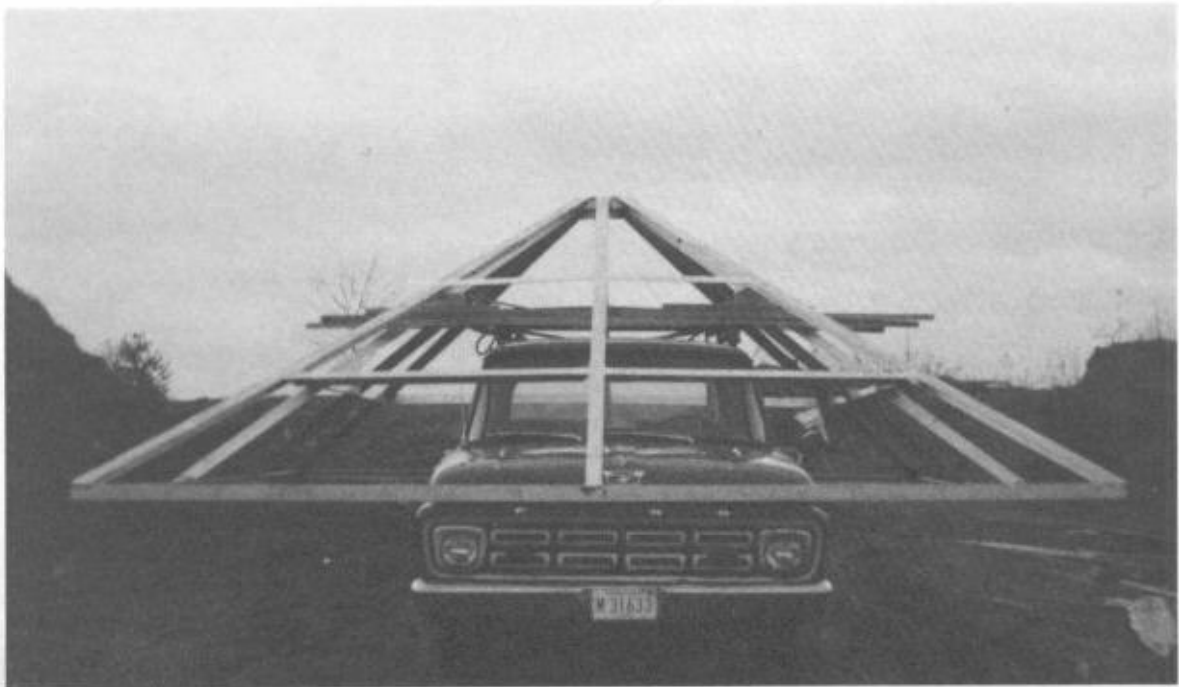
Fig. 18-12. Not the approved way of moving a skylight frame, but it worked.
